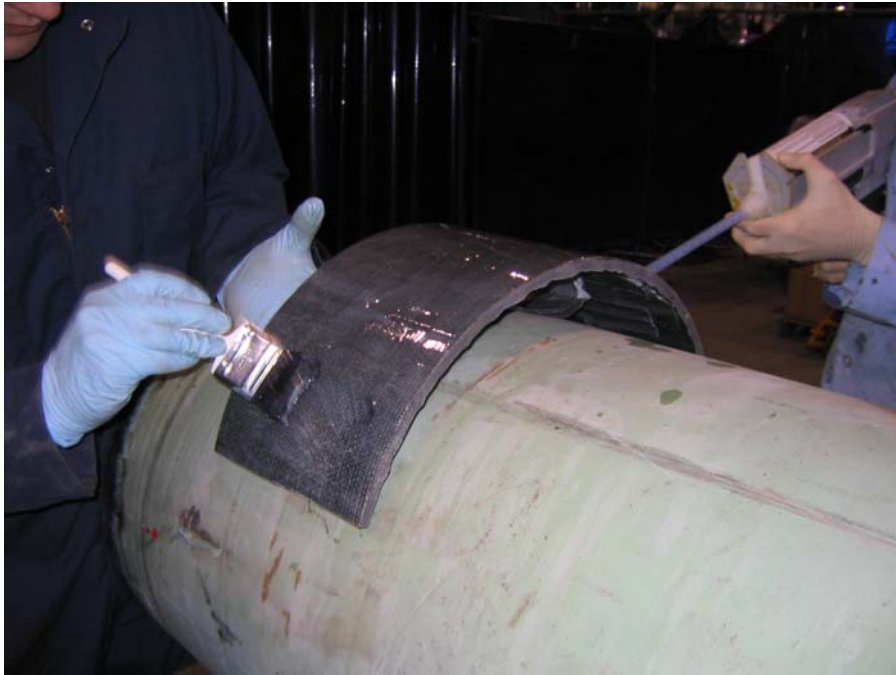
Figure 24 - Application of Adhesive to Repair Patch
