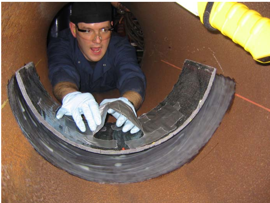
Figure 25 - Installation of Repair Patch
