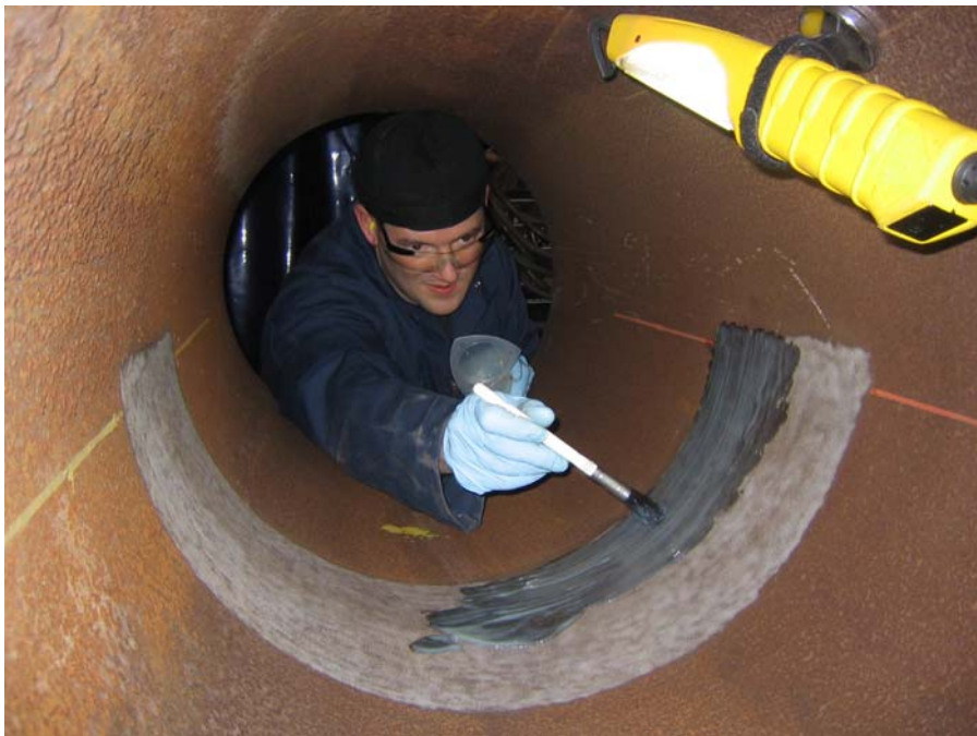
Figure 23 - Application of 3M DP460 Adhesive to Grit-Blasted Inside Diameter of Pipe
