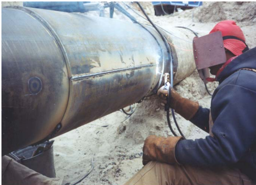
Figure 1 - Installation of a Full-Encirclement Repair Sleeve
