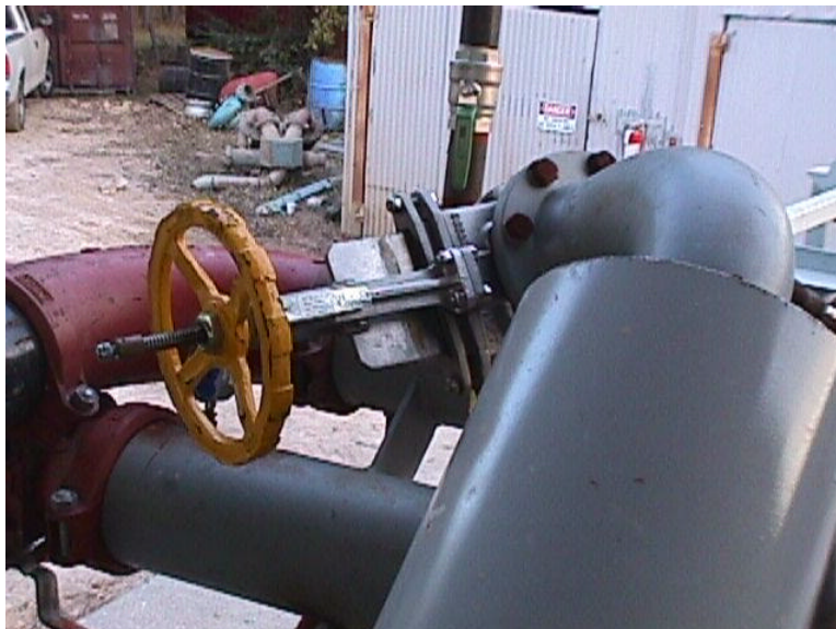
Figure 62. Adjustment Gate Valve
