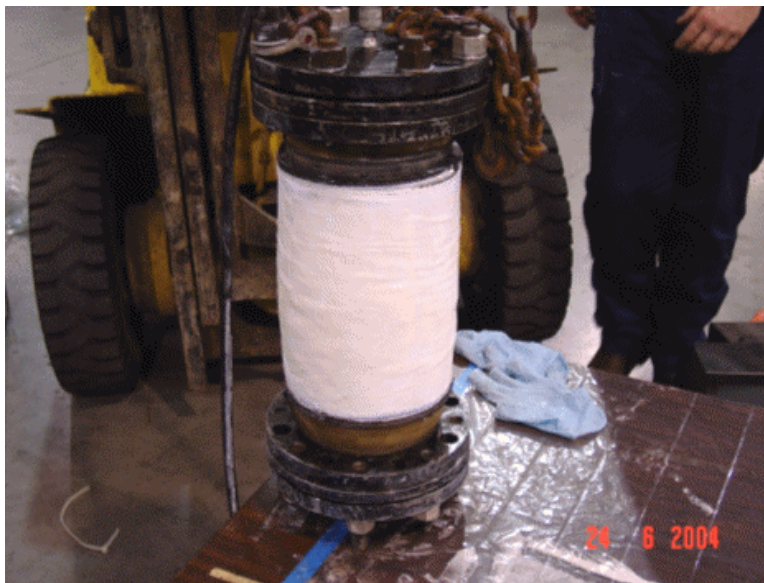
Figure 8. Repair Sleeve with Epoxy Applied
