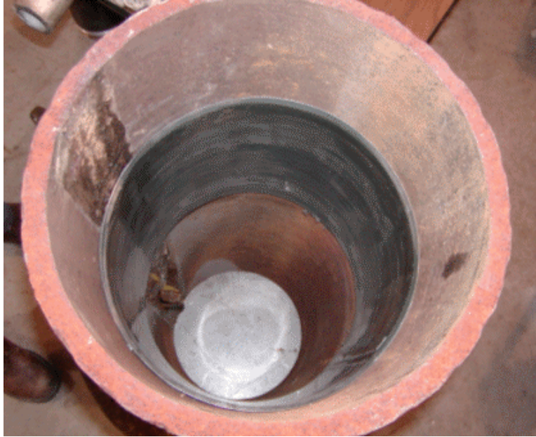
Figure 11. Successfully Installed Repair Sleeve
