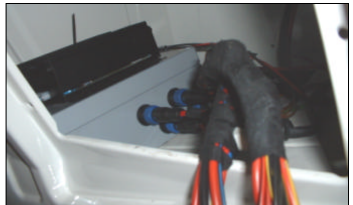
Figure 17 - Installation of System Control Unit on VW LT35 Van
