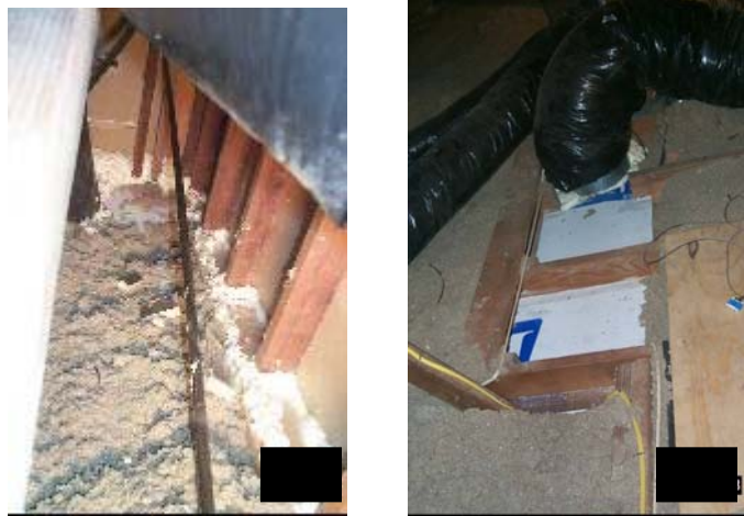
Figure 3. Sealing cavities connecting the house to the attic. Foam was used for sealing small holes and cracks at building component intersections (left). Duct board insulation was used to block off large open areas (right)
