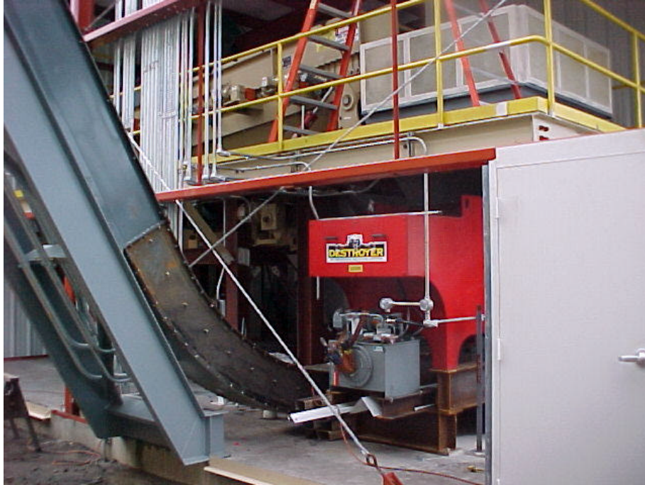
Figure 3. Construction Picture Showing Installation of Disc Screen (above), Grinder (below) and Conveyor from Screening to the Walking Floor Bin
