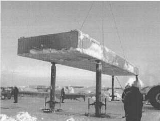
Figure A-3. Setting the First Platform Module
