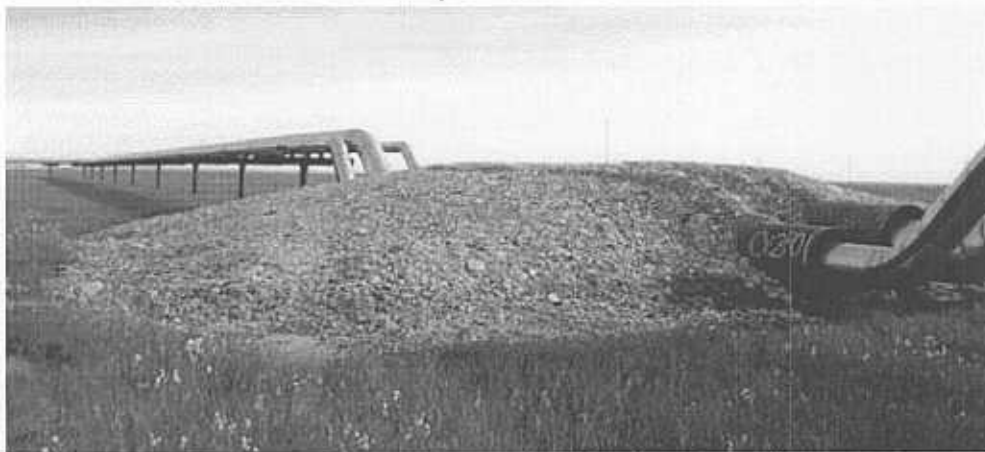
Figure 8. Gravel Ramp for Pipeline Crossing
