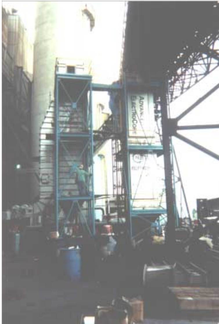
Figure 18: Assembled Precharger and Advanced ElectroCore Module
