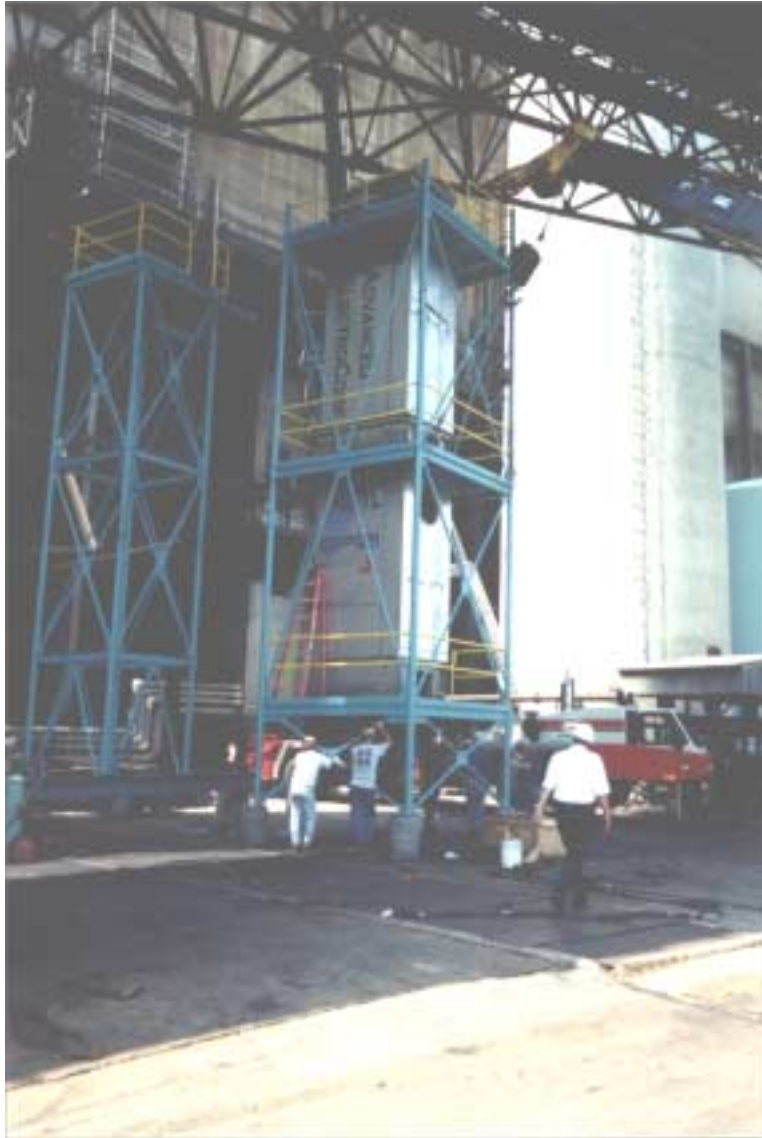
Figure 16: Advanced ElectroCore Module in Place on Foundations
