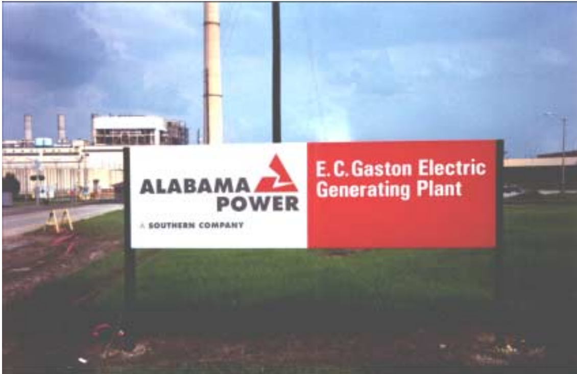
Figure 12: Advanced ElectroCore Installation Site in Wilsonville, Alabama
