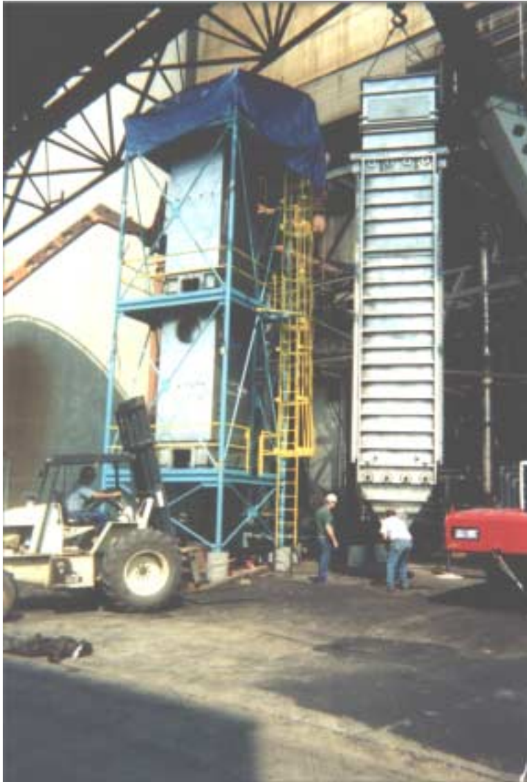
Figure 17: Precharger Being Lifted Onto Precharger Support Frame
