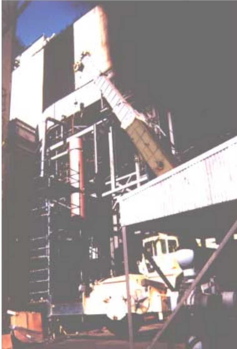
Figure 19: Dry Scrubber Being Lifted and Set in Place on Concrete Foundation
