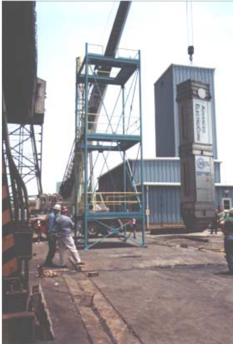
Figure 15: Advanced ElectroCore Module Ready to be Inserted Into its Support Frame
