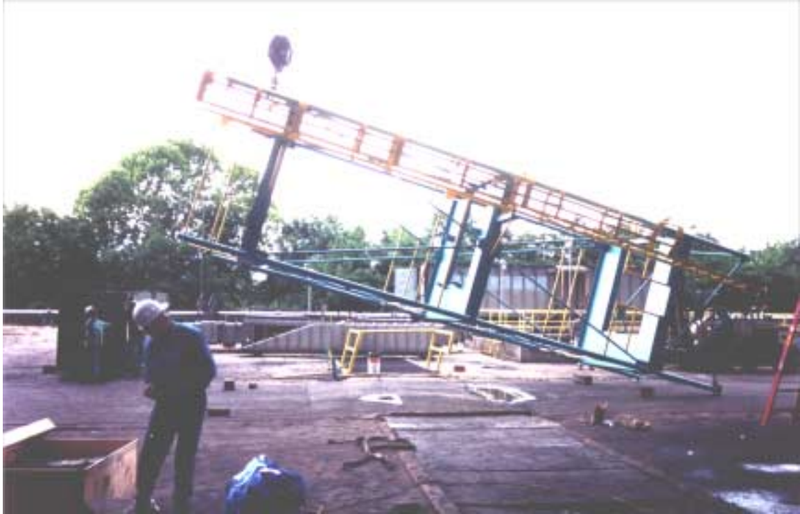
Figure 13: Standing Up the Advanced ElectroCore Module Support Frame
