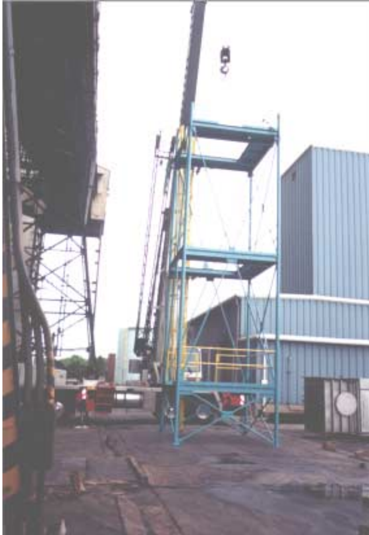
Figure 14: Advanced ElectroCore Module Frame Erected
