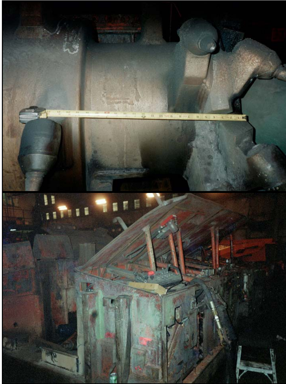
Figure 5.27. View of the SUFCO 12CM12 during rebuild. The photos here show the eventual mounting locations for the HS-CM display enclosure and sensor enclosure. The actual installation took place underground at SUFCO and no photos are available.
