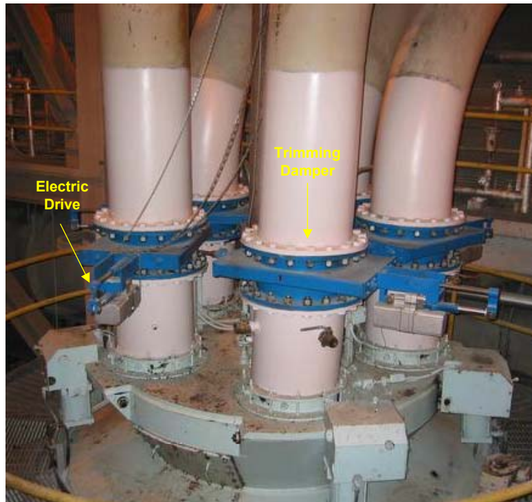
Figure 2-19. Photograph of damper installation.
