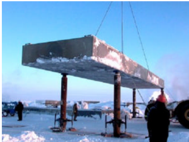
Figure A-3. Setting the First Platform Module
