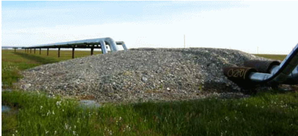
Figure 8. Gravel Ramp for Pipeline Crossing
