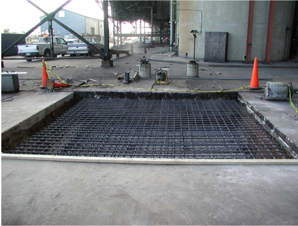
Figure 1. Foundation excavation and supporting rebar just prior to pouring concrete, Gaston January 2003.
