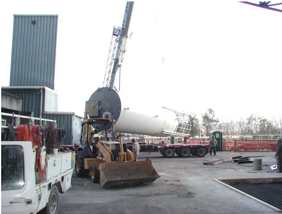
Figure 2. Lifting the carbon silo from the truck before setting on the foundation, Gaston January 2003.
