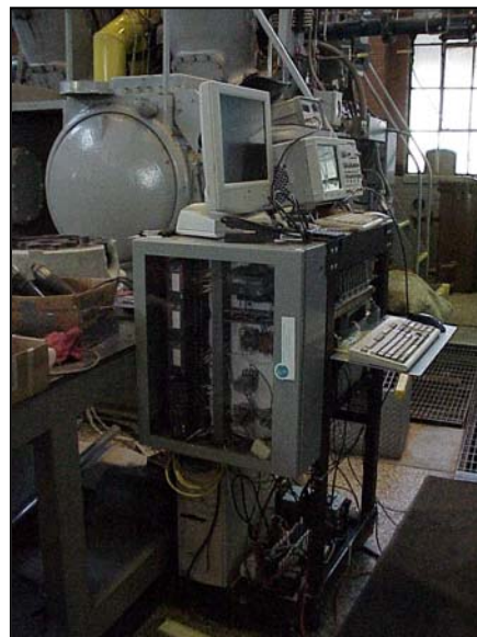
Figure 3. Micropilot control system for engine operation
