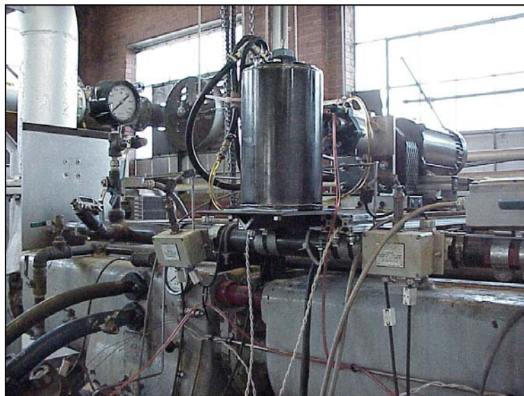
Figure 4. Pilot fuel pump and storage mounted on GMV test engine
