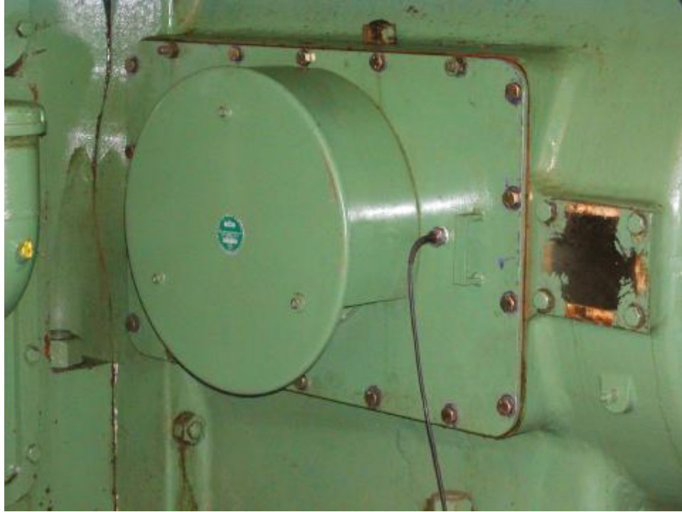
Figure 6. Cable from RLM Antenna
