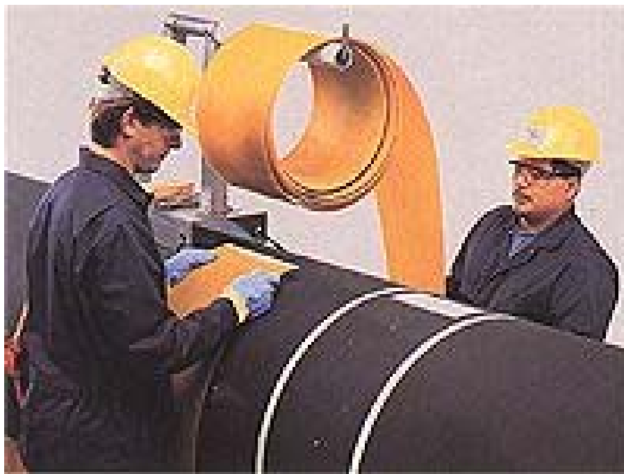
Figure 4 - Clock Spring® Fiber-Reinforced Composite Device for Pipeline Repair
