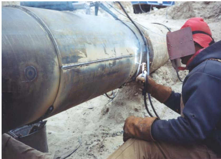
Figure 1 - Installation of a Full-Encirclement Repair Sleeve
