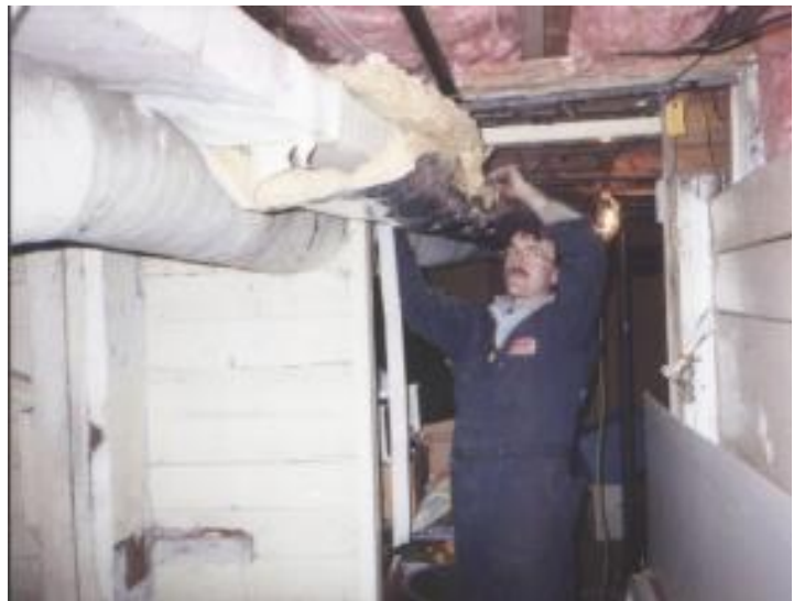
Installing Duct Wrap
