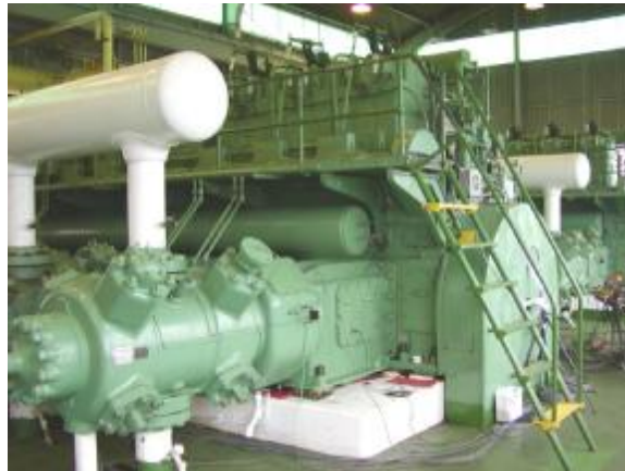
Figure 1. Initial Site Test (HBA-6, TGP Kinder Station)
