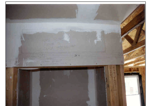
AHU closet. Note continuous air barrier over doorway in foreground. Installers cut a tightly tolerated opening here for the main supply trunk which blocked access to the chase
