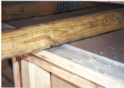
Top of chase from attic. Leakage path down interior wall (after supply run outs are installed).
