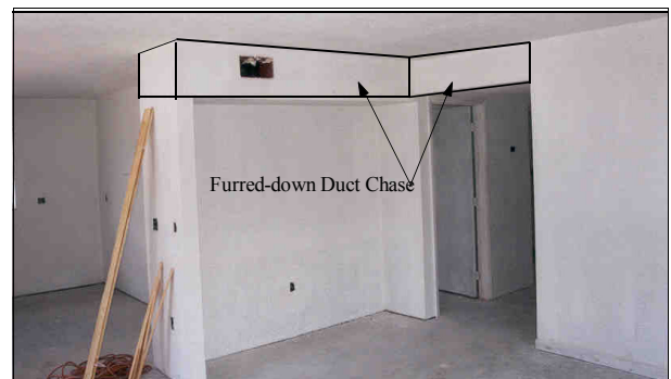
Figure 1 Hallway furred down duct chase continues out into living space creating an alcove. Broward County Habitat for Humanity.
