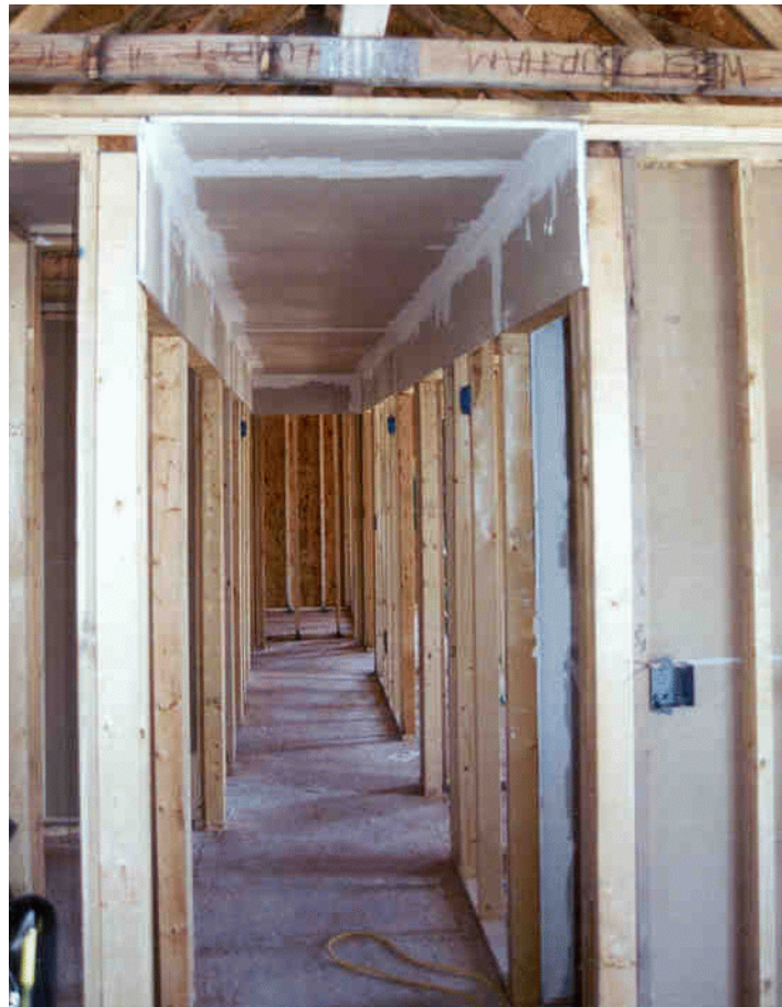
North Carolina construction. From living area looking down the hall toward bedrooms. Hallway fur down with drywall air barrier sealed at the seams and edges with drywall mud.
