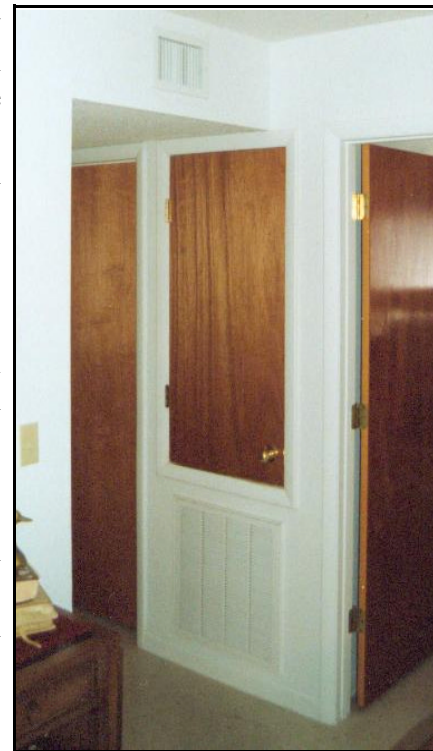
Figure 7 Interior air handler closet with return under a platform dividing the closet. Lakeland Habitat for Humanity, Central Florida.
