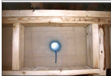
Supply register location. Note absence of seal at top plate to chase side.
