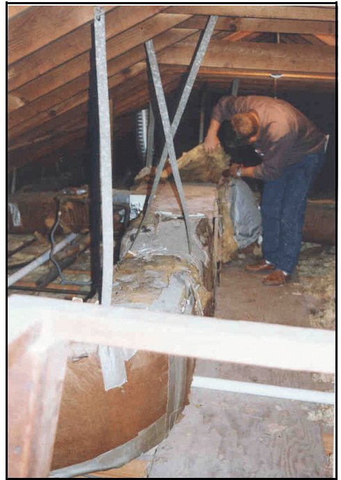
Figure 3 Ducts and air handlers in unconditioned spaces where supply leakage can create conditions ideal for condensation, mold growth, and building decay.
