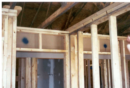
Back of chase side seen from bedroom. Registers are marked with blue spray paint
