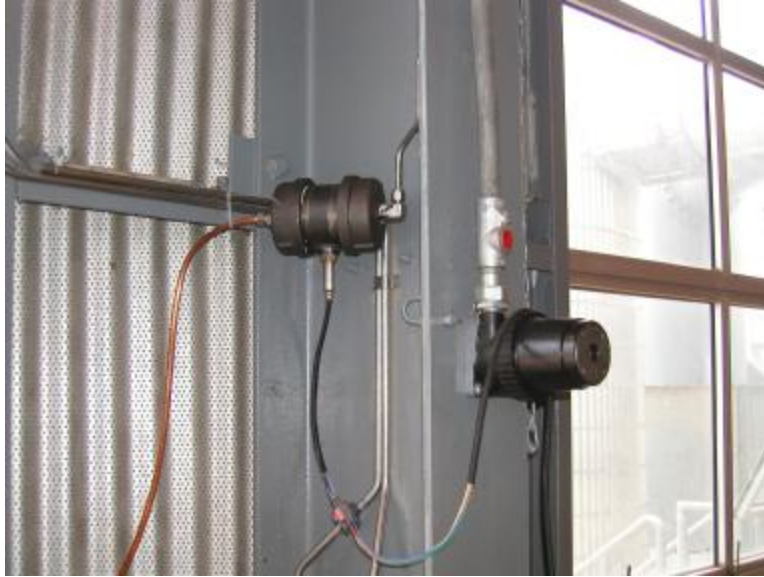
Figure 19. O 2 /NO x Sensor and Connection to Line from Stack (GMW10, Williams Sour Lake Station)
