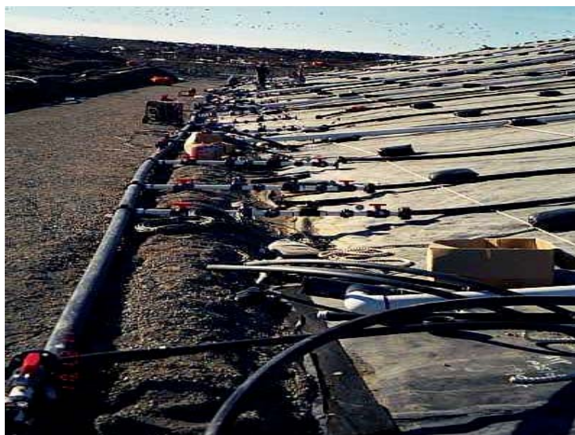
Image 3-7. Leachate injection header and laterals
