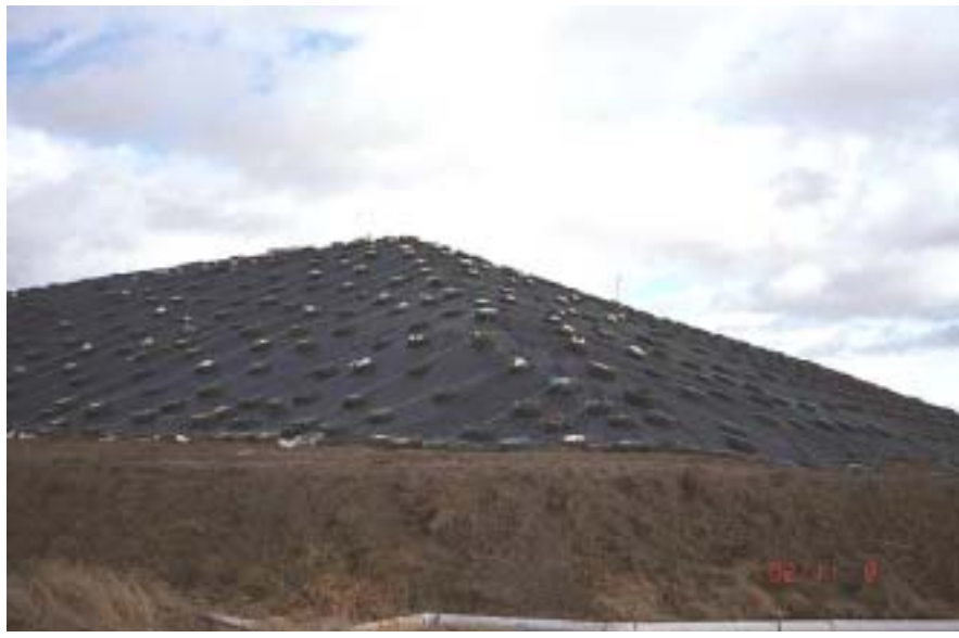
Image 4-4. West-side anaerobic cell surface liner.
