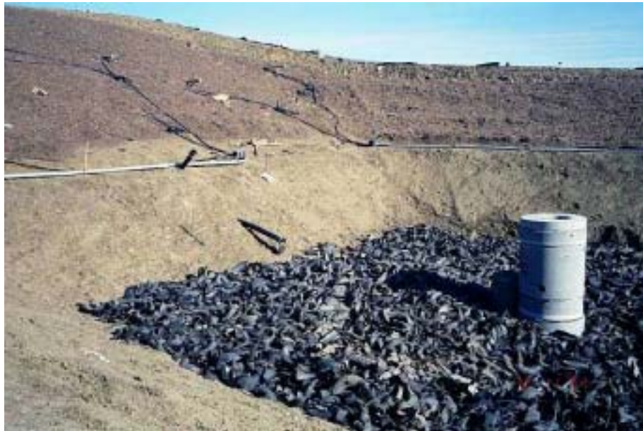
Image 5-8. Aerobic sump installed and ready for backfill
