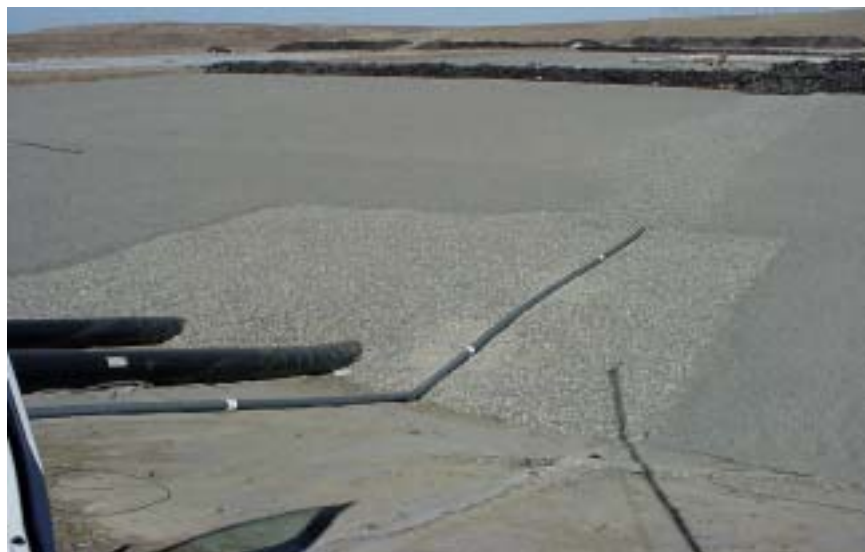
Image 3-5. Gravel drainage layer and leachate collection sump
