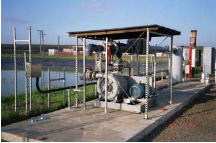
Image 5-3: Aerobic Cell Blower Station
