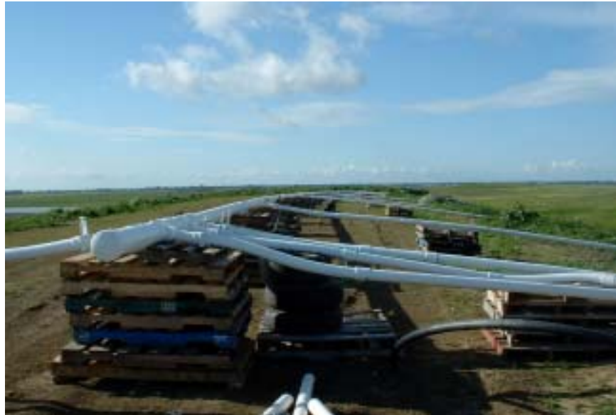
Image 4-3. LFG collection laterals connected to the main header line located on top the cell.
