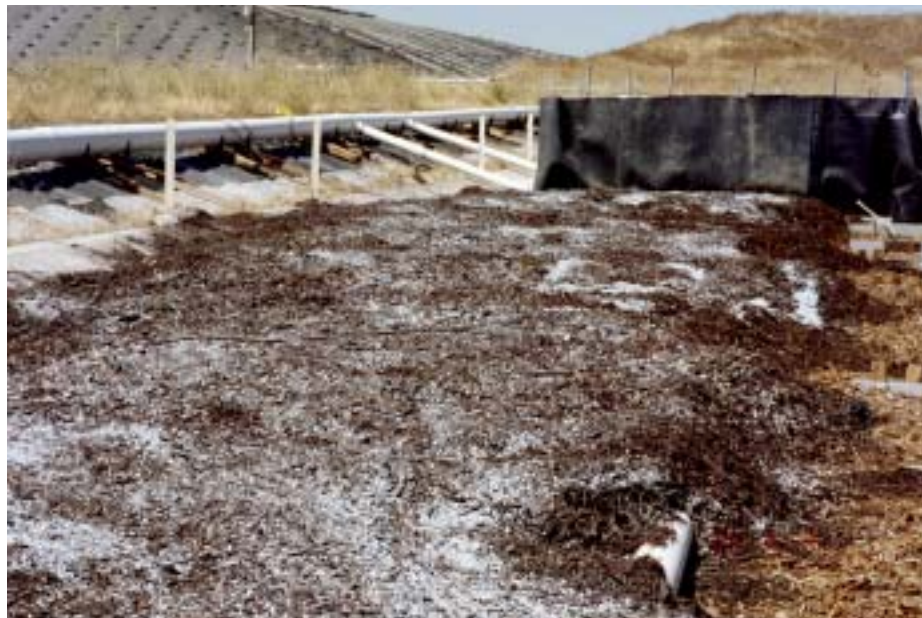
Image 5-6. Limestone sprinkled on the first lift of the biofilter.
