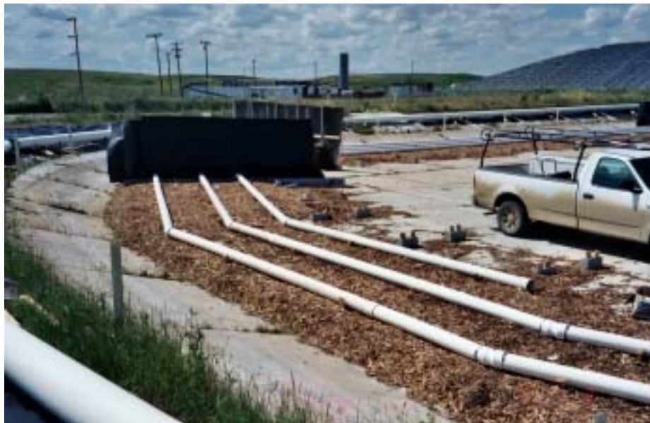
Image 5-4. Biofilter base with piping installed.
