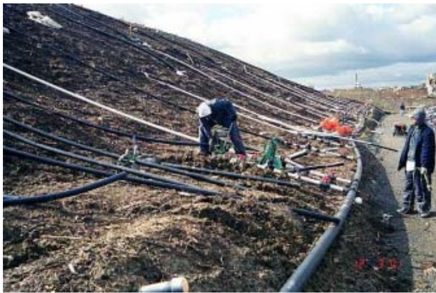
Image 5-9. Aerobic leachate injection header and lateral
