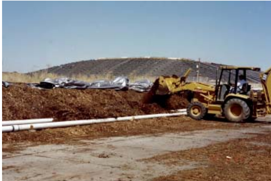
Image 5-5. Placement of biofilter media.
