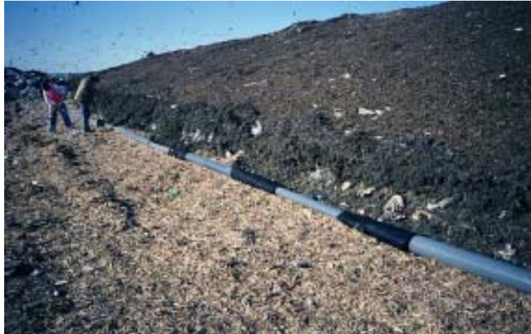
Image 3-2. Horizontal LFG collection line
