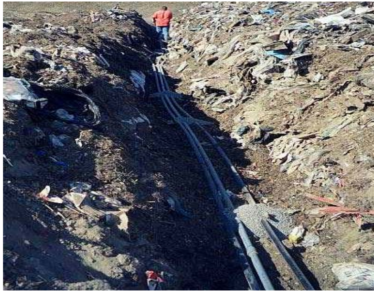
Image 5-2. Leachate injection laterals in trench
