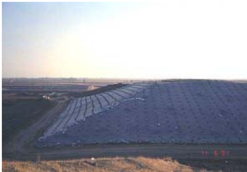
Image 3-3. Northeast anaerobic surface liner
