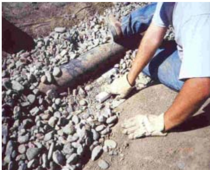
Image 6-2. Pressure tubes installed in LCRS trench
