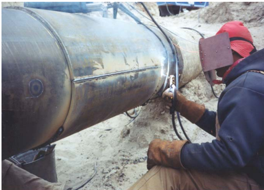
Figure 1 - Installation of a Full-Encirclement Repair Sleeve
