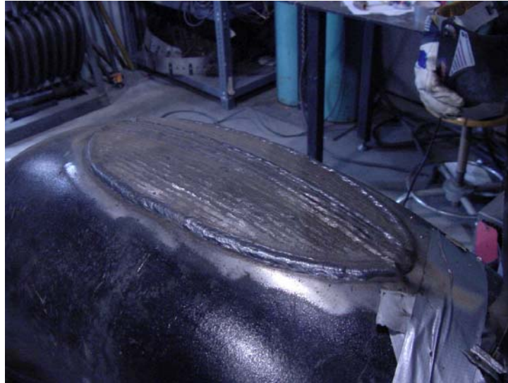
Figure 2 - External Weld Deposition Repair of Internal Wall Loss in 90 Degree Elbow
