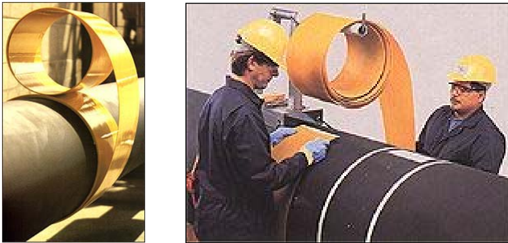
Figure 4 - Clock Spring® Fiber-Reinforced Composite Device for Pipeline Repair
