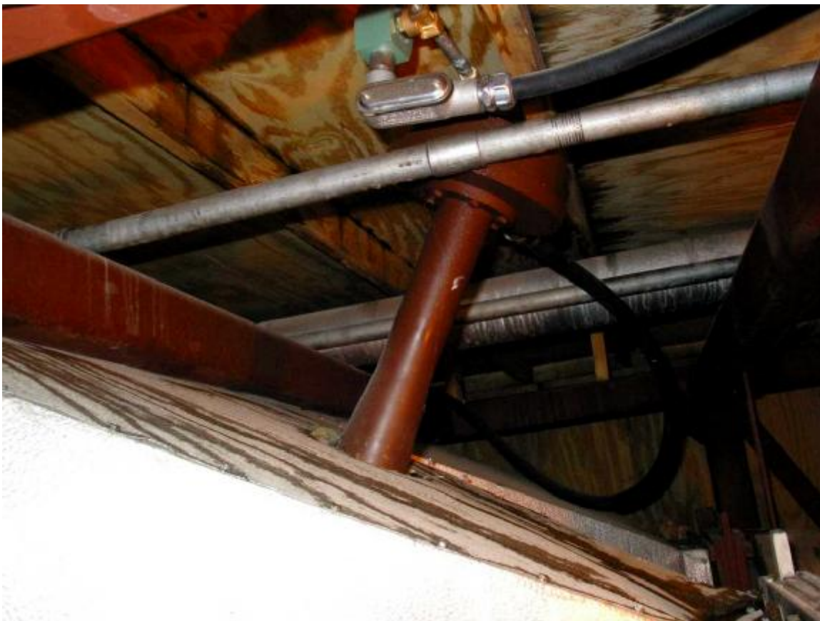
Figure 3. Typical Sonic Horn Installation on the Pilot Unit at CCS.
