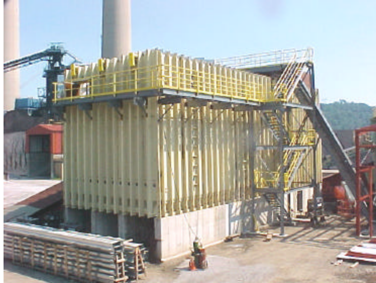
Figure 8. The Keith Mfg. Walking floor bin under construction
