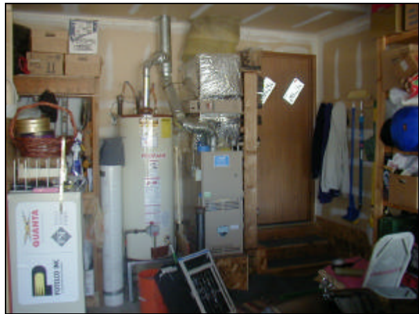
Figure D-10. Gas furnace in garage.
