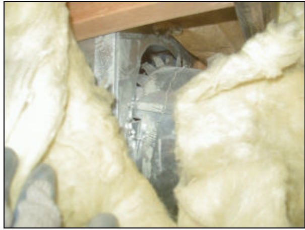
Figure D-14. Leak at supply plenum.
