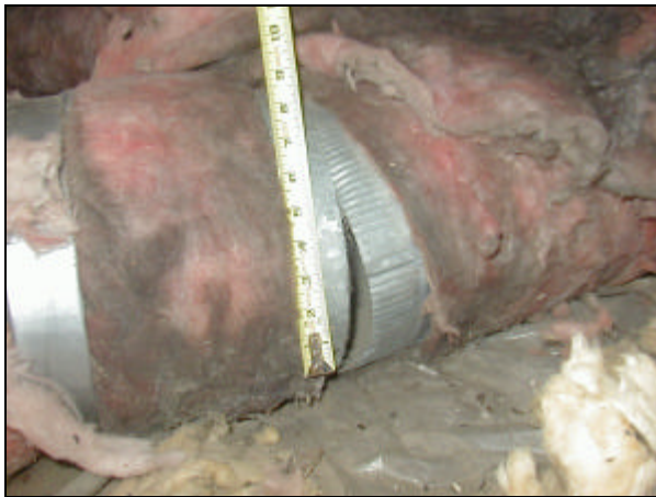
Figure D-15. Separated supply duct.
