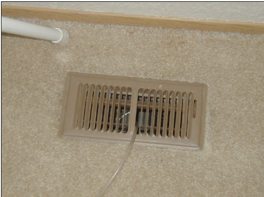
Figure 2-13. Typical floor register.
