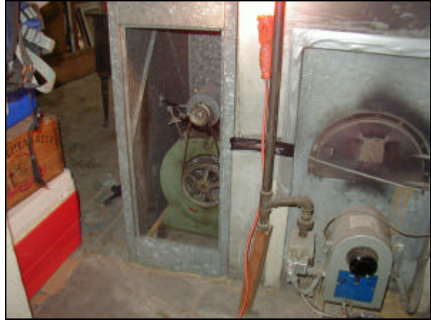
Figure D-8. Old converted furnace, belt-driven.
