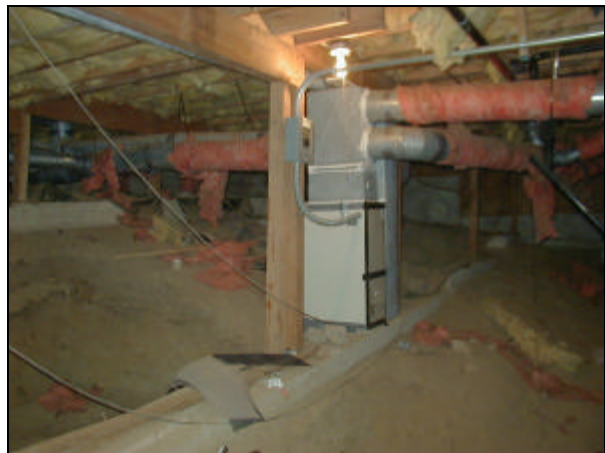
Figure D-12. Furnace in high crawl space.
