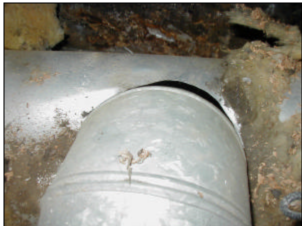
Figure D-18. Supply duct coming out of trunk.
