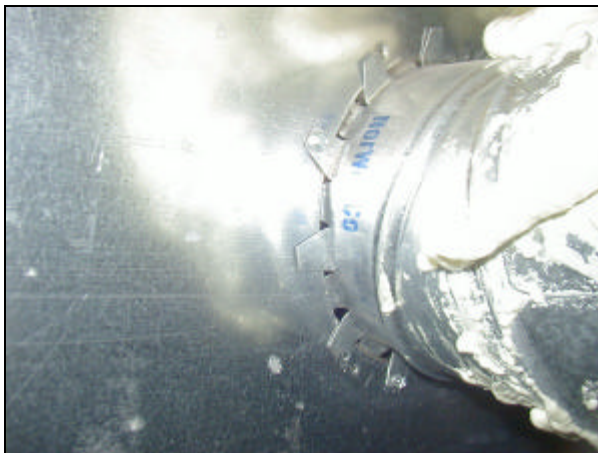
Figure D-17. Leaky finger joints.
