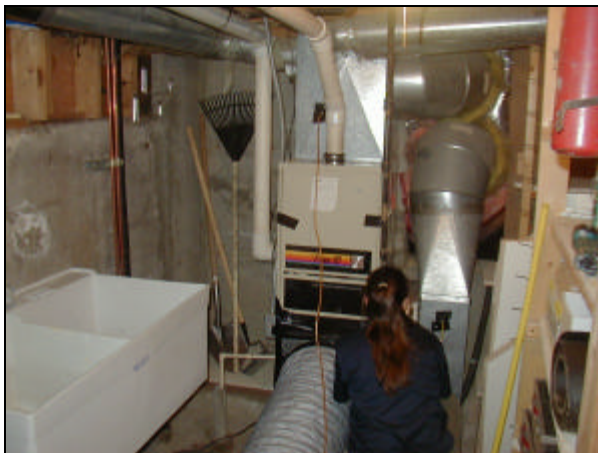
Figure D-11. New condensing gas furnace.
