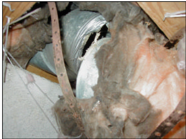
Figure D-16. Separated elbow at supply boot.
