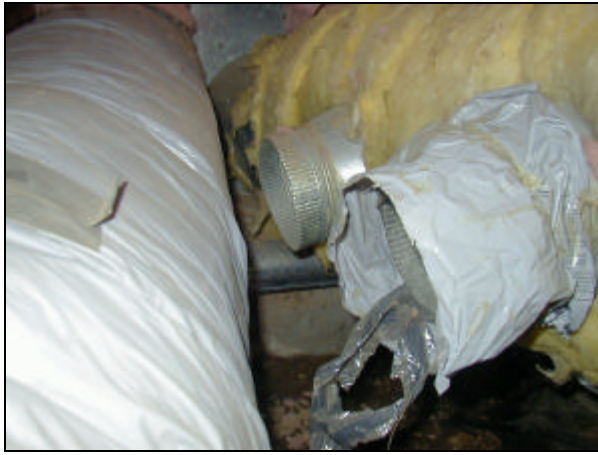
Figure D-13. Double disconnected supply.
