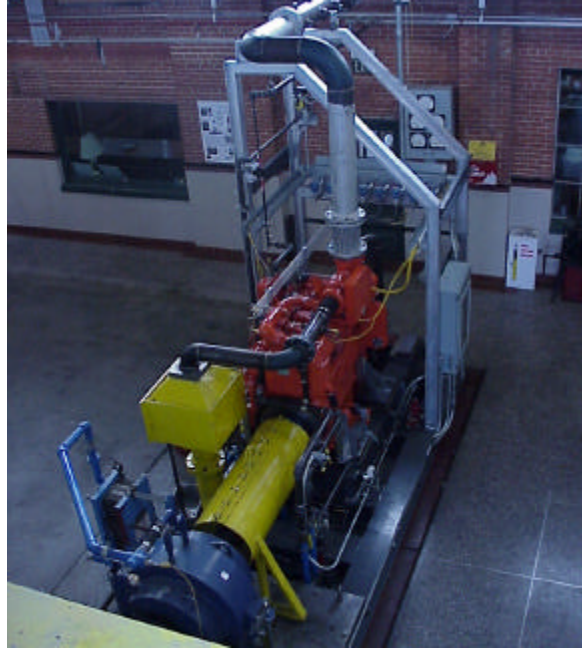
Figure 14: Installation of Waukesha F18 Natural-Gas Engine at CSU
