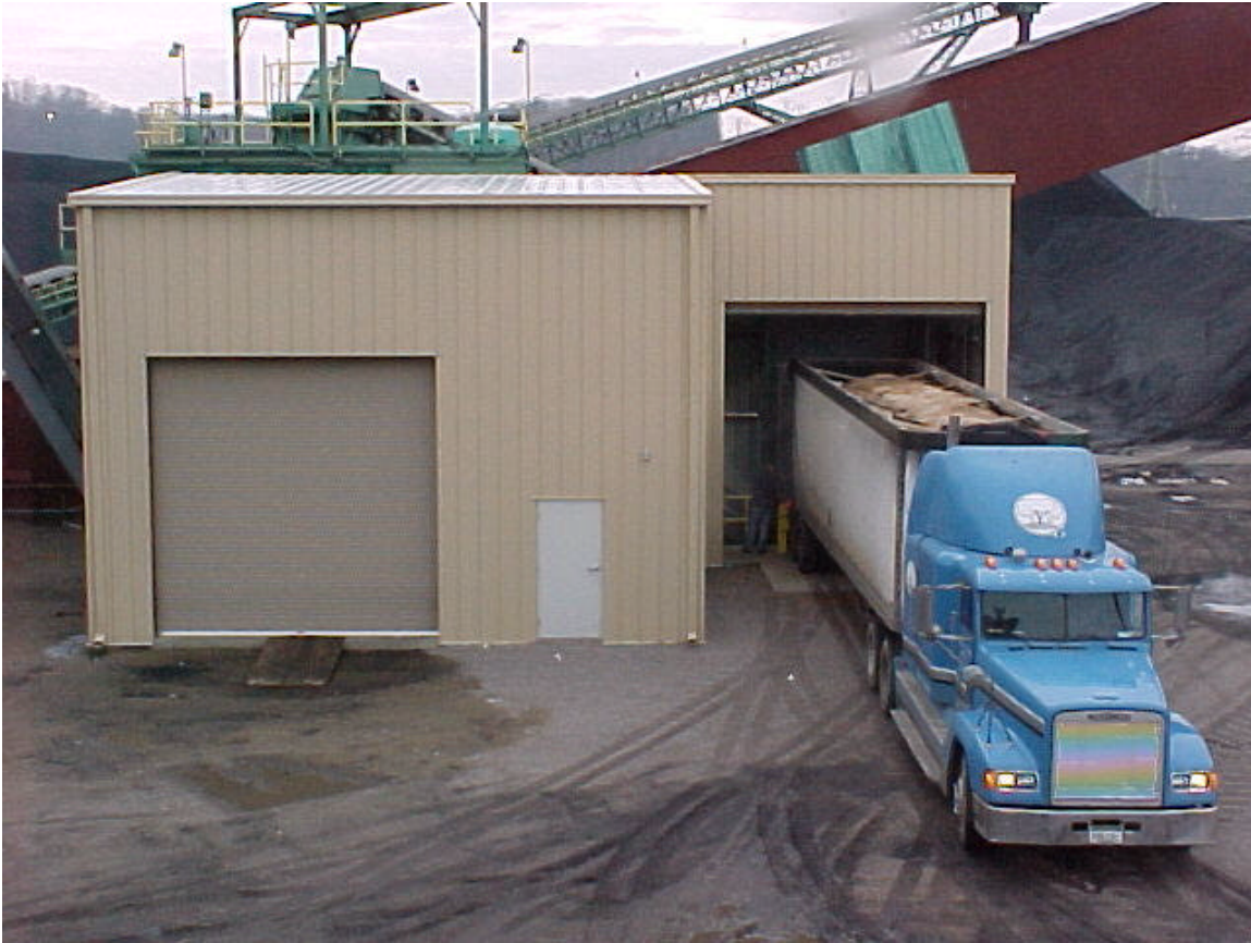
Figure 2. Cofiring Installation at Willow Island Generating Station. This installation includes fuel receiving, screening, and grinding of oversized particles in the main building (shown), and fuel storage, reclaim, and metering (to the main belt) in the walking floor bin (not shown).
