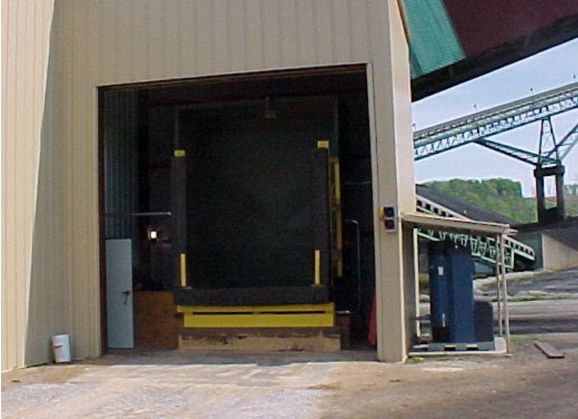
Figure 1. The improved sawdust receiving system including plexiglass barriers and dock seals.
