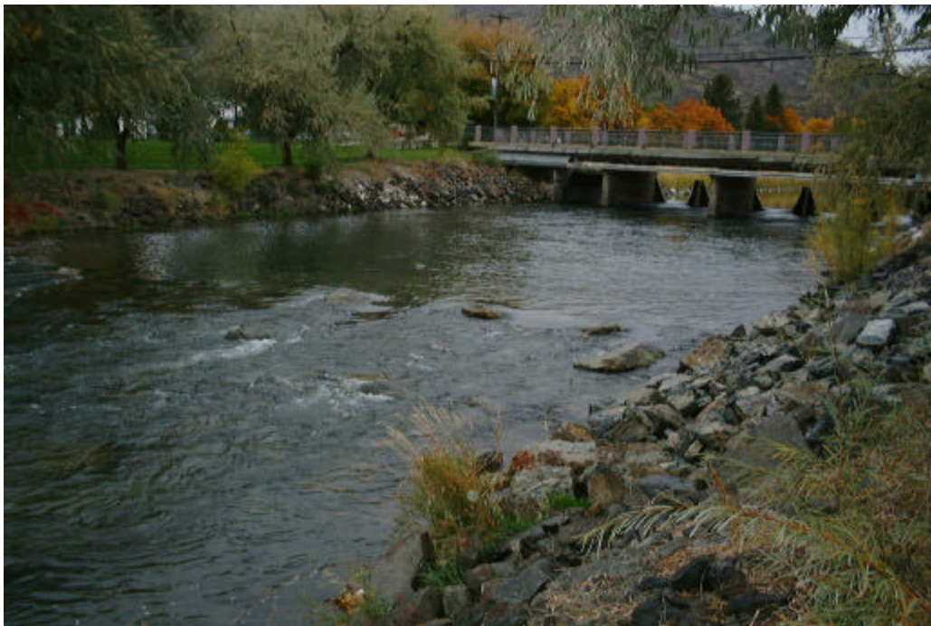
Figure 4-6: the fall below drop structure 12 is distributed over four riffles constructed in 2001. The drop at the structure is less than 15 cm, allowing easy fish passage upstream and downstream.
