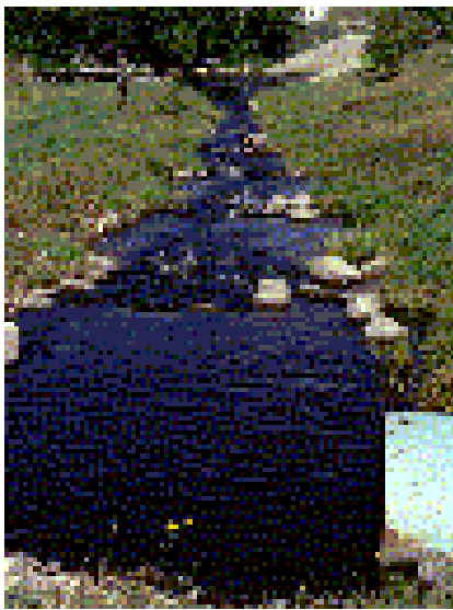
Figure 4-9: typical pool and riffle fishway on the earthfill portion of the Rapid City dam, MB. The channel leads from the tailrace to a pool and im[pounded culvert (foreground) that is connected to the forebay through a gated entrance.
