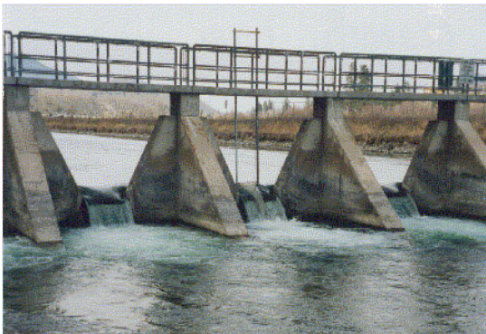
Photo 16: concentrated fall below drop structure 14 in potential spawning Reach C.
