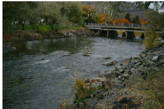
Photo 17: the fall below drop structure 12 is distributed over four riffles constructed in 2001. The drop at the structure is less than 15 cm, allowing easy fish passage upstream and downstream.
