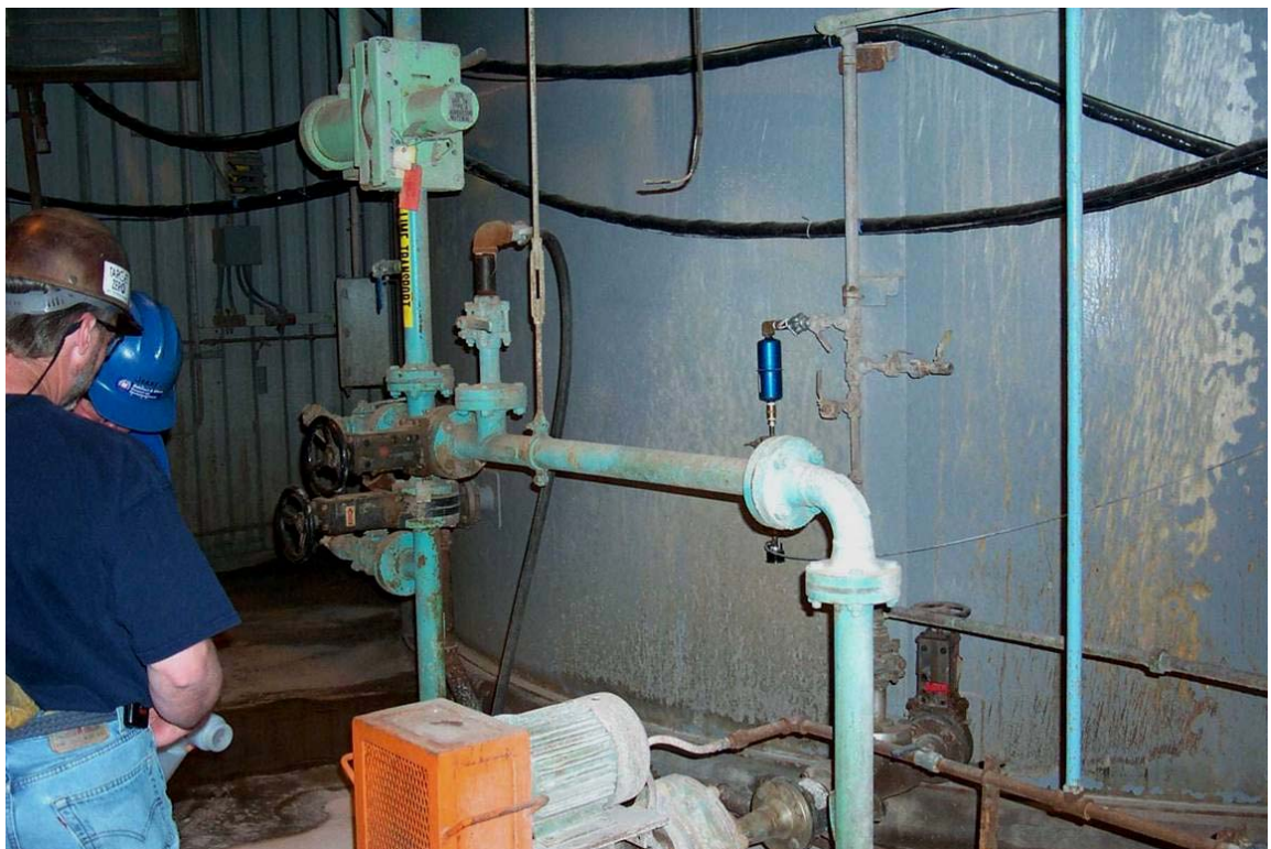
Figure 3.5-6: Limestone Slurry Pump and Storage Tank at Endicott
