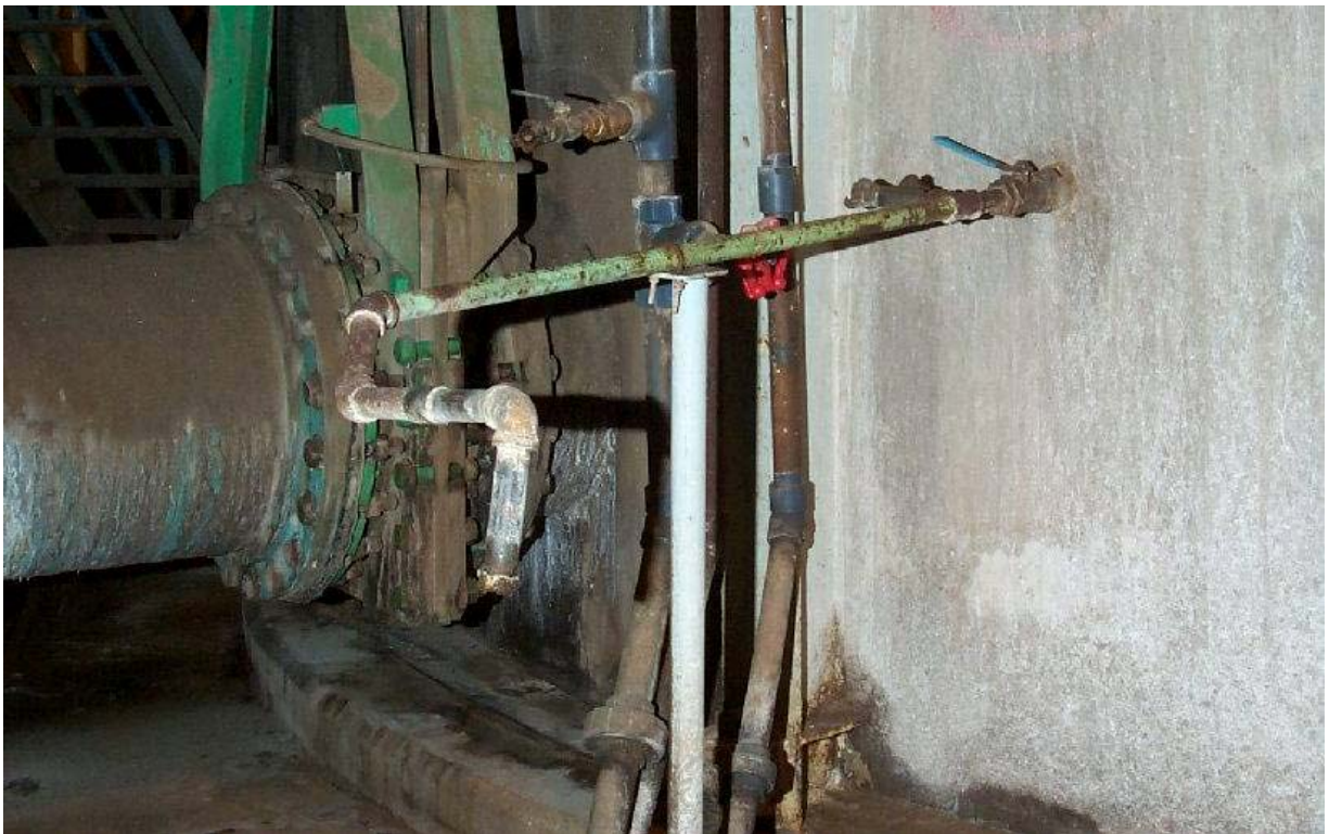
Figure 3.5-10: Wet FGD Slurry Sample Tap on the Absorber Recirculating Tank at Endicott
