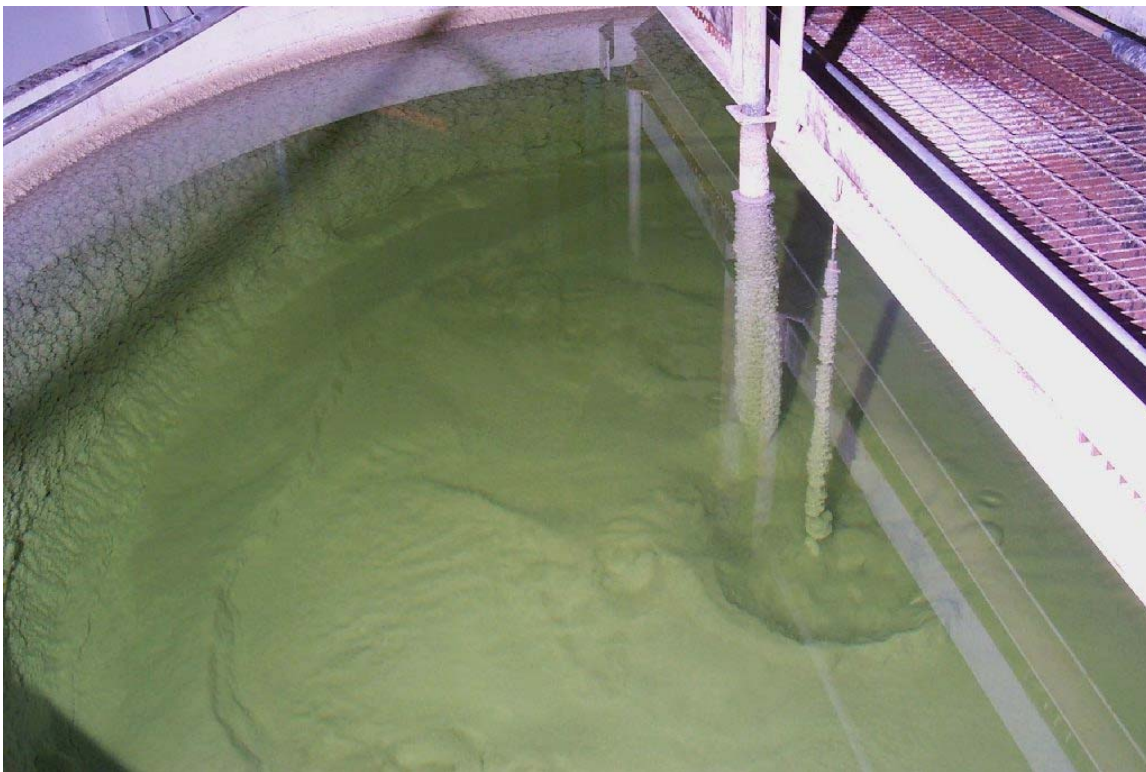
Figure 3.5-7: Settled Sludge in a Tank in the Water Treatment Process at Endicott
