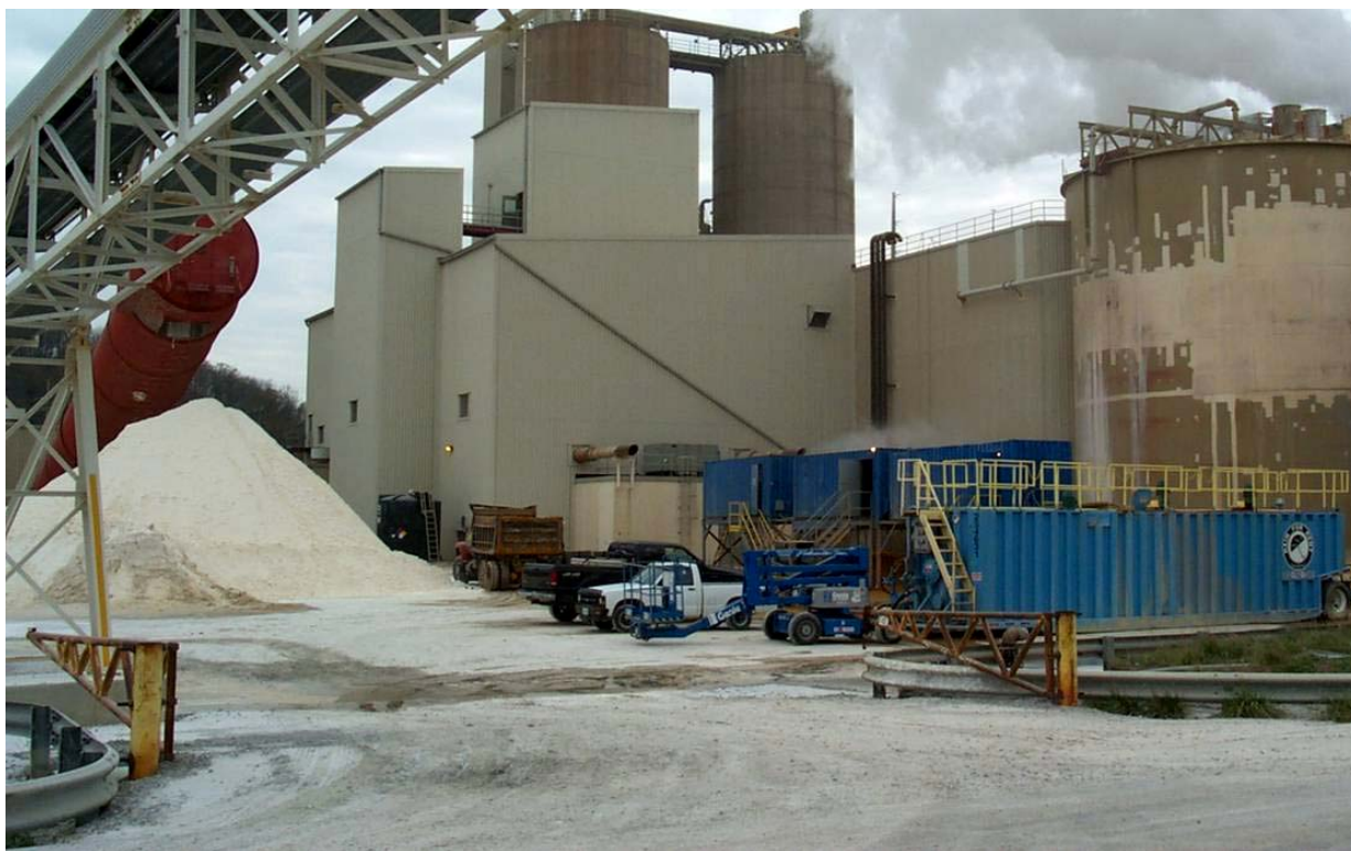
Figure 3.5-21: Gypsum Pile (left, white) and Centrifuges (center, blue) at Zimmer
