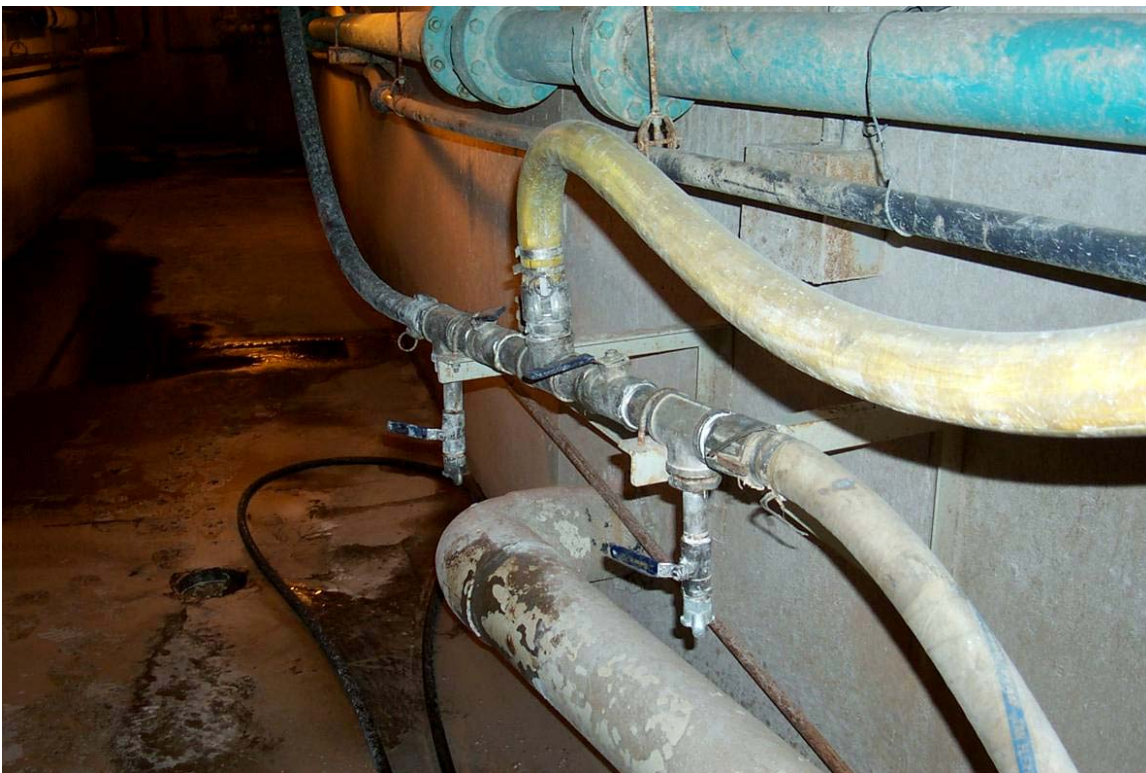
Figure 3.5-8: Sample Point for the Water Treatment Sludge at Endicott
