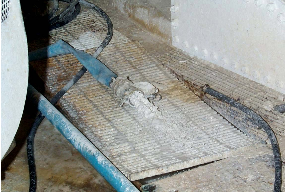
Figure 3.5-13: Thiosorbic Lime Slurry flowing from Storage Tanks at Zimmer
