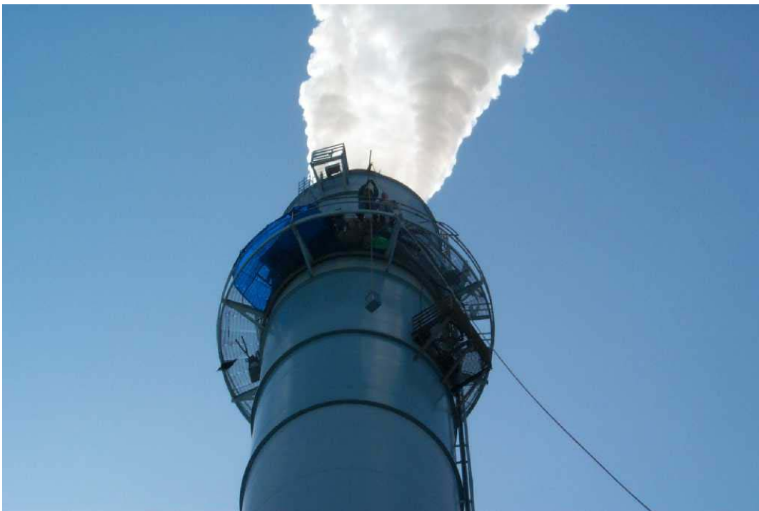
Figure 3.3-2: Wet FGD Outlet (Stack) Sampling Location - Endicott
