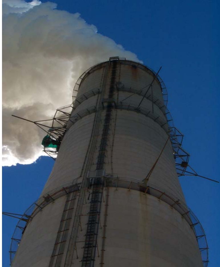
Figure 3.3-13: Wet FGD Outlet Sampling - Zimmer
