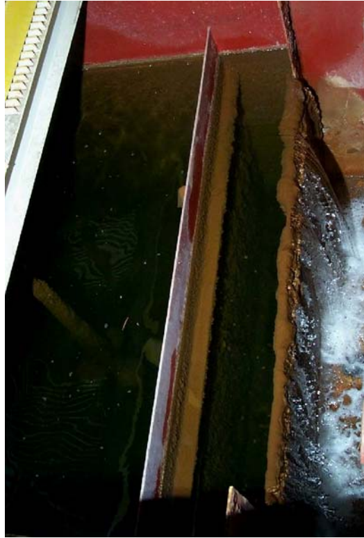
Figure 3.5-9: Treated Water Overflow Weir at Endicott
