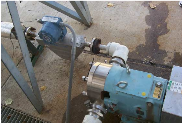
(b) Variable frequency pump (0~2000GPM)
