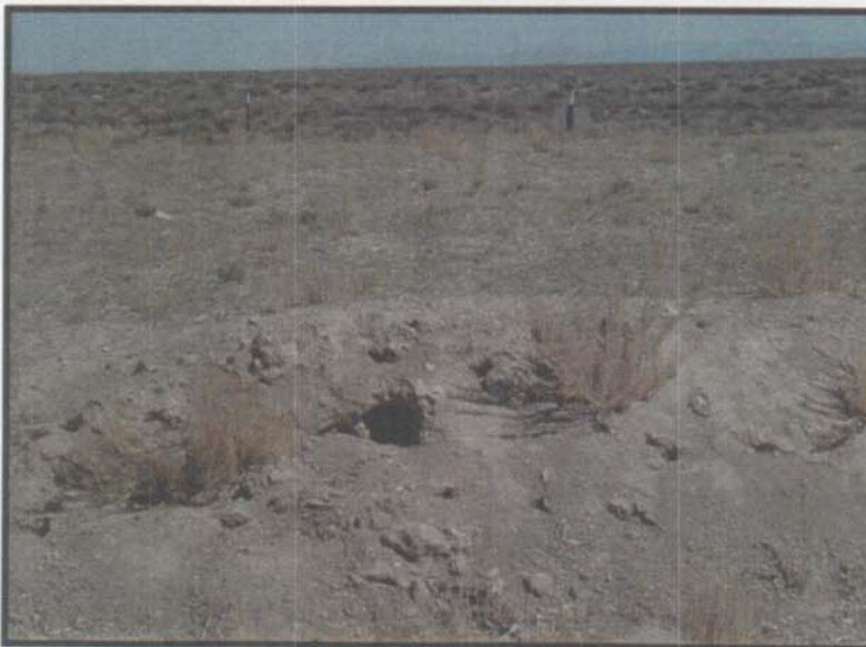
Animal burrows along edge of cover cap at the Roller Coaster RADSAFE area.
