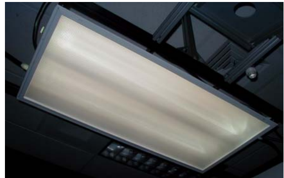
Fig. 8 - Mounted Hybrid Luminaire with Fiber Optic and Fluorescent Sources On
