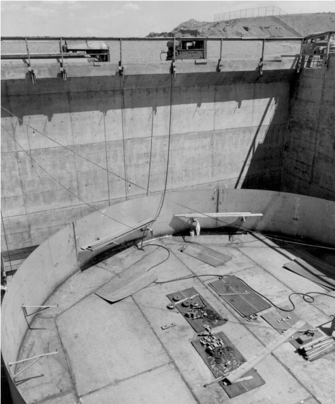
Figure D-1. Construction of Tank WM-188 (58-3473).
