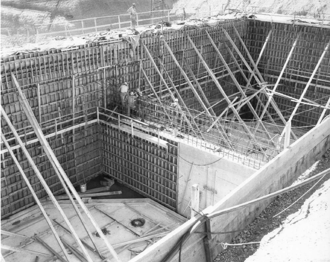
Figure 6. Square, poured-in-place vaults for Tanks WM-189 and -190, and the type used for Tanks WM-187 and WM-188 (63-4240).
