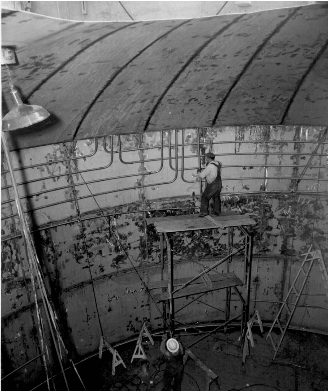
Figure D-3. Installation of cooling coils for Tank WM-187 (58-4237).
