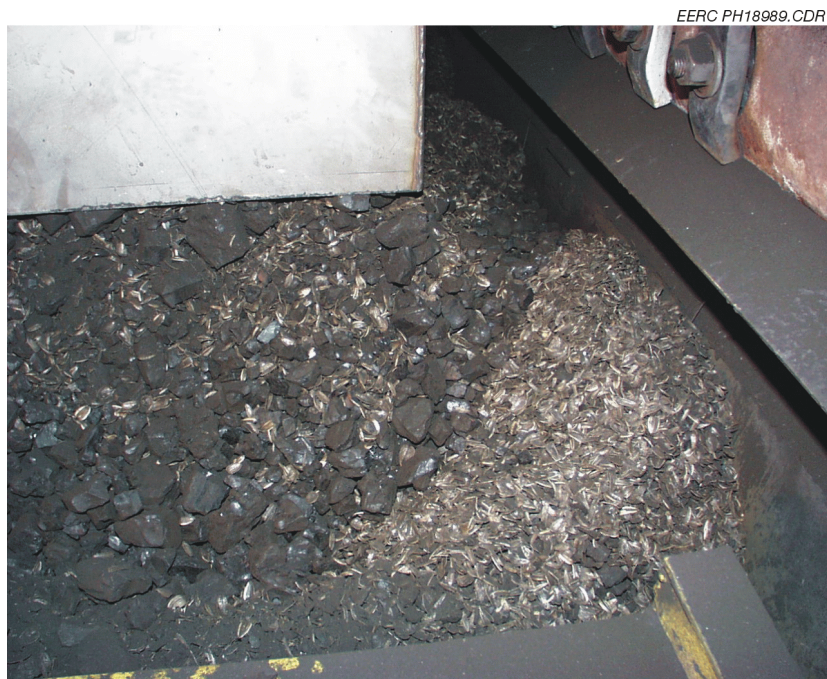
Figure 8. Example of segregation issue at stoker inlet on Boiler No. 3.
