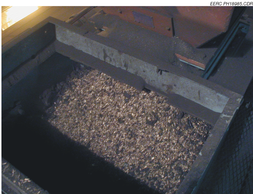
Figure 5. Fuel feed at discharge of bunker on Boiler No. 5 prior to stokers.
