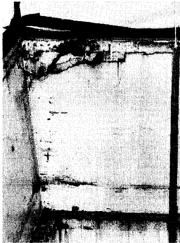
Figure 6-1. Damage Caused By Coverblock.
