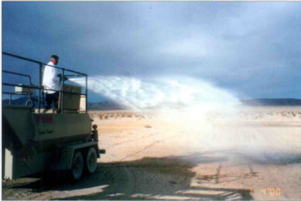
Figure 3-29. Applying tackifier with a hydroseeder.
