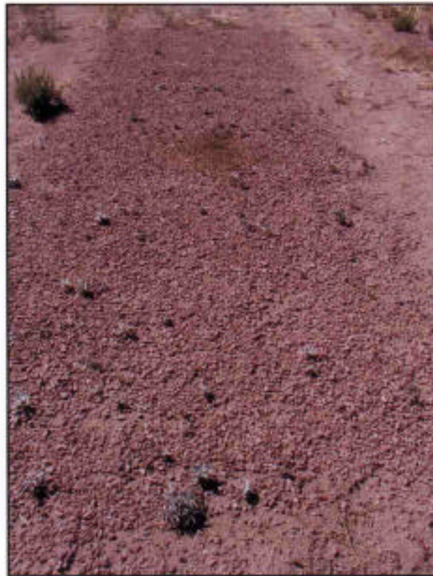
Figure 3-5. Example of gravel armoring (1.5 cm in diameter) used to control erosion.
