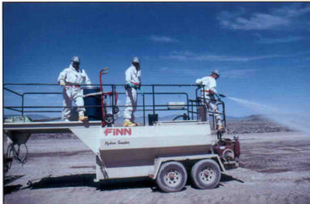
Figure 3-6. Applying chemical soil stabilizer with a hydromulcher.
