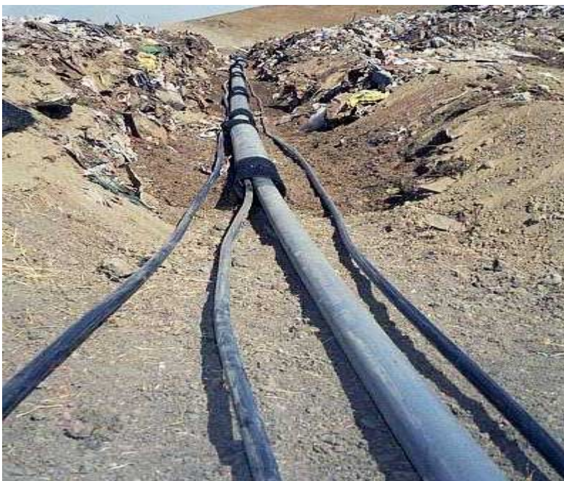
Image 10: Horizontal air collection line
