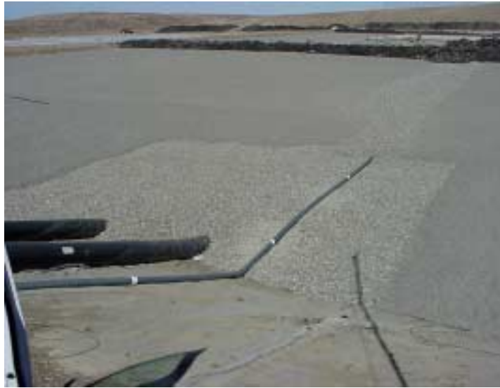
Image 5: Gravel drainage layer and leachate collection sump
