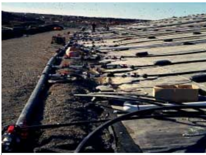
Image 6: Leachate injection header and laterals
