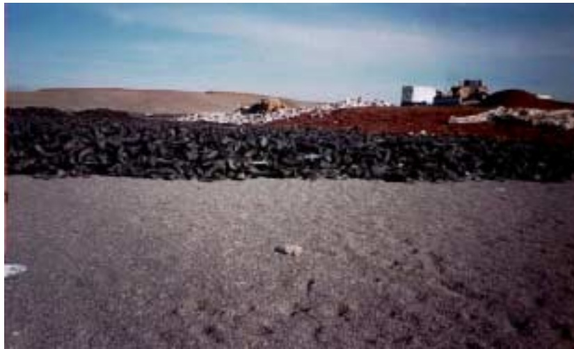
Image 14: Shredded tire operations layer
