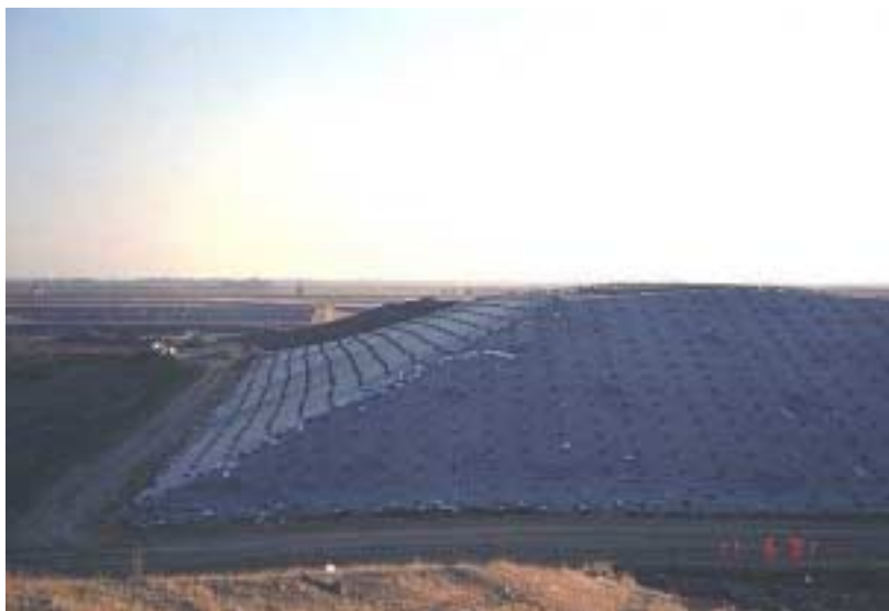
Image 3: Northeast anaerobic surface liner
