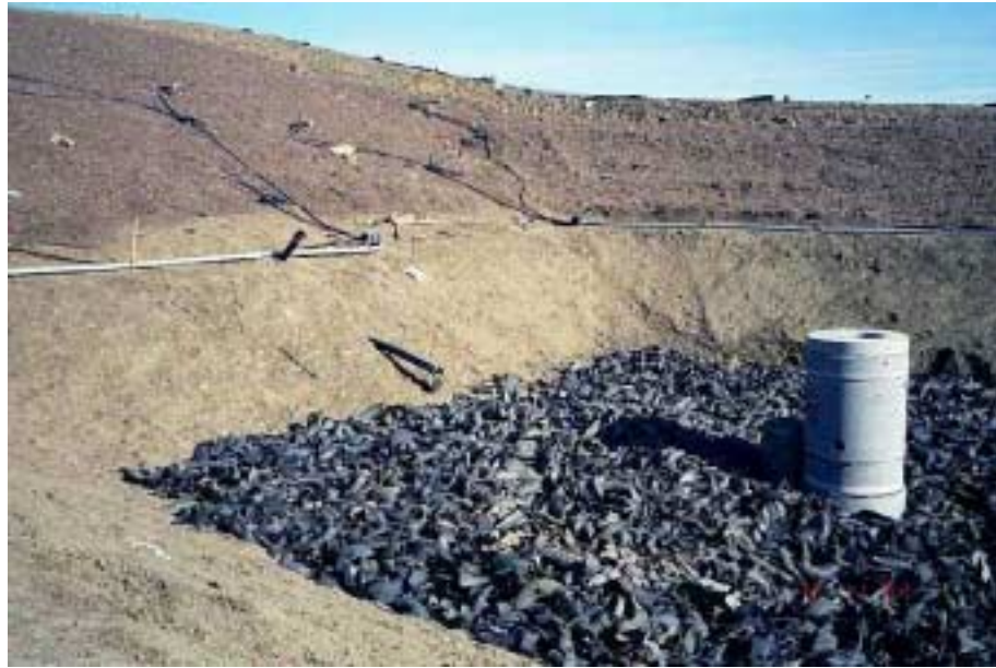
Image 12: Aerobic sump installed and ready for backfill
