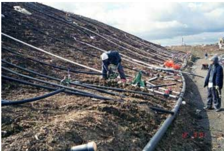
Image 13: Aerobic leachate injection header and lateral
