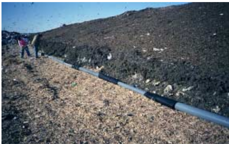
Image 2: Horizontal LFG collection line installation
