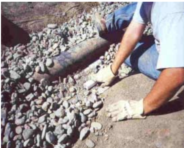
Image 15: Pressure tubes installed in LCRS trench
