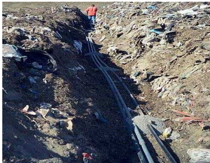
Image 9: Leachate injection laterals in trench
