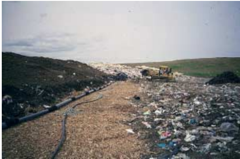
Image 1: Horizontal LFG and leachate injection lines installed and being covered by shredded tires.
