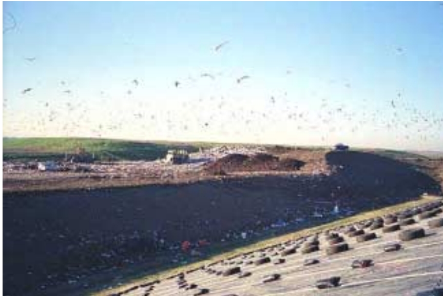
Image 7: Waste placement in the west-side cell
