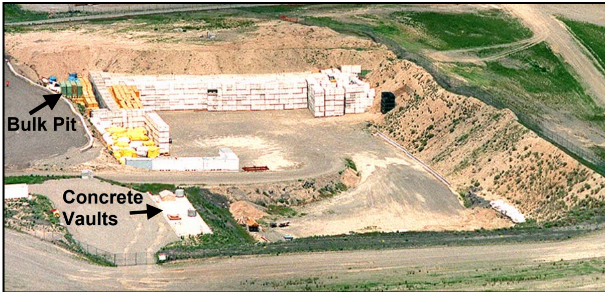
Figure 3. Photo of currently operating LLW disposal pits within the SDA.
