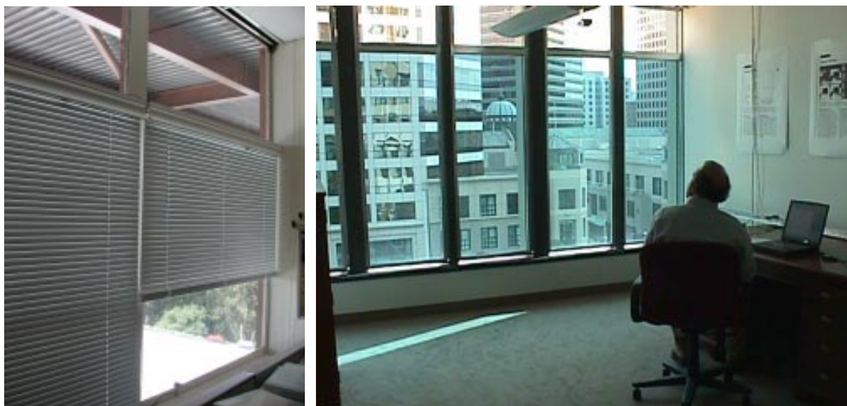
Figure 2. Automated Venetian Blind System based on Dallas Semiconductor 1-Wire® (left) and Large-Area Electrochromic Windows in Oakland Federal Building with Windows in Bleached on Top and Colored State on Bottom (right).
