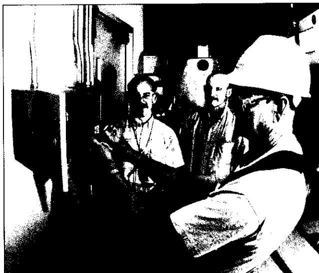
Time meters are installed to measure operating hours of the crane in the background.
