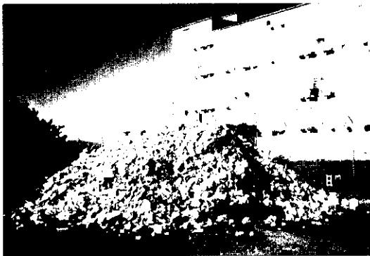
The concrete rubble was transported to the 100B and C sites where it was used to fill in areas where contaminated soil was excavated during cleanup.
