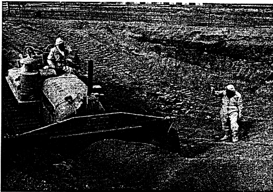
Photo 175-03-TTR-63 shows Radiological Control Technicians during the Roller Coaster Followup Operation directing a bulldozer operator during digging for buried debris at the Rad Safe Waste Pit at Tonopah
