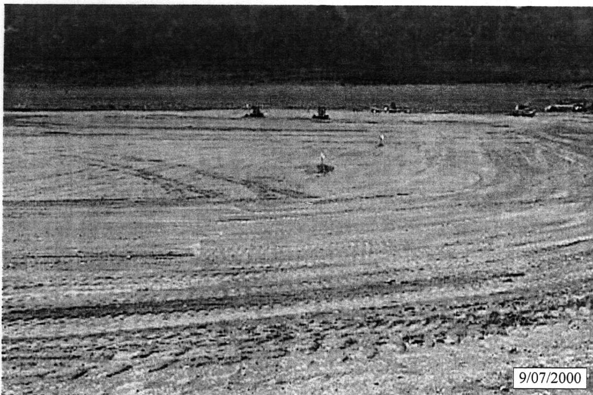
PHOTOGRAPH 14 - Completed 4 foot earthen mono-layer CMP cover
