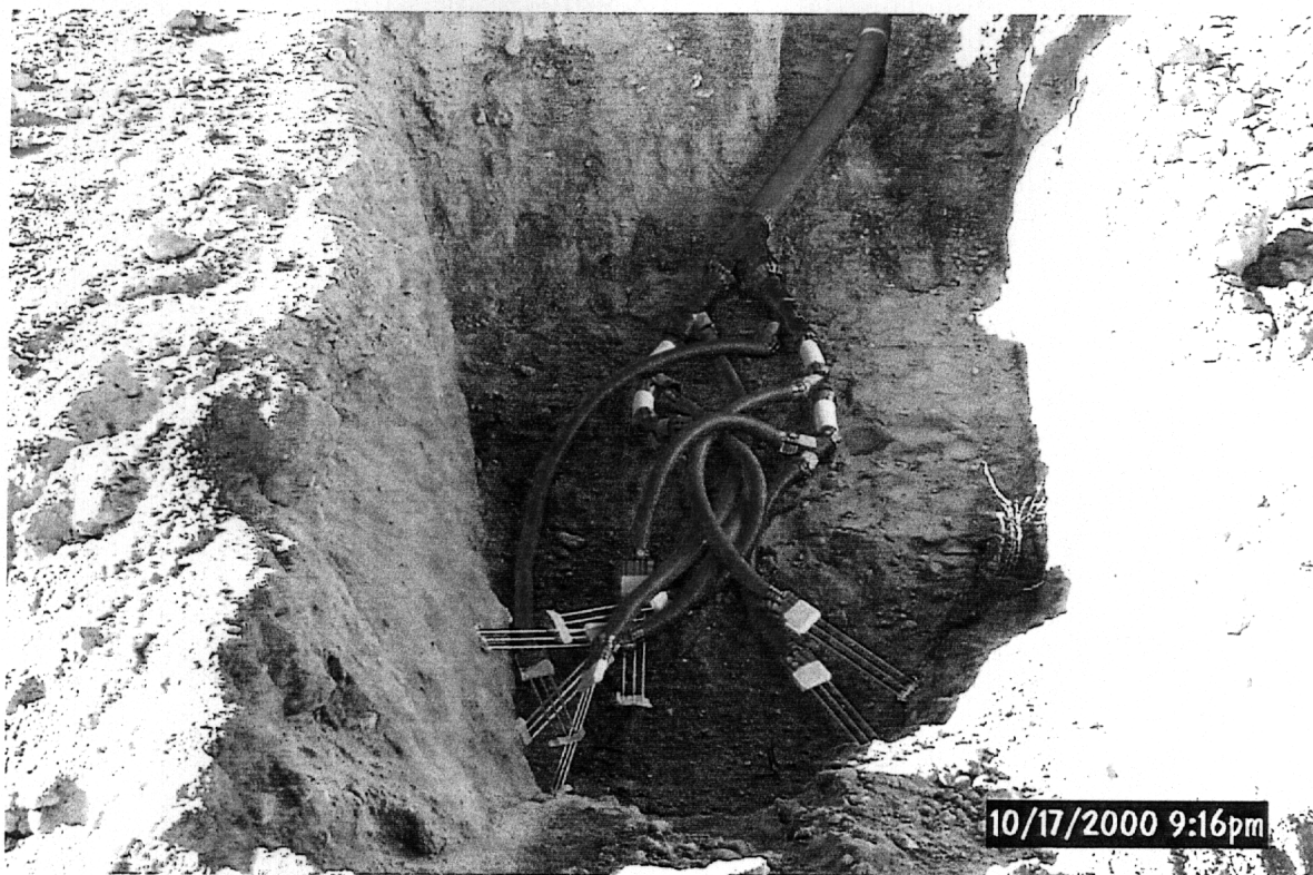
PHOTOGRAPH 21 - Installing TDR sensors in CMP cover
