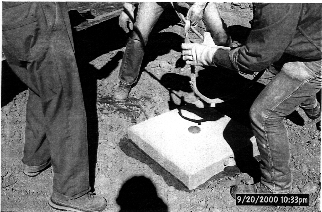
PHOTOGRAPH 20 - Placing subsidence monuments on the CMP cover
