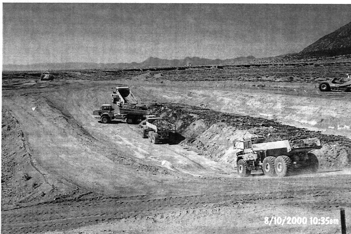
PHOTOGRAPH 8 - Drilling material from UC-4 Area S being placed in Relocation Trench
