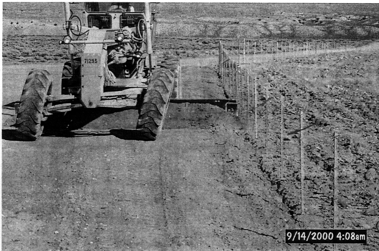
PHOTOGRAPH 18 - Burring the wire mesh "bunny" fencing
