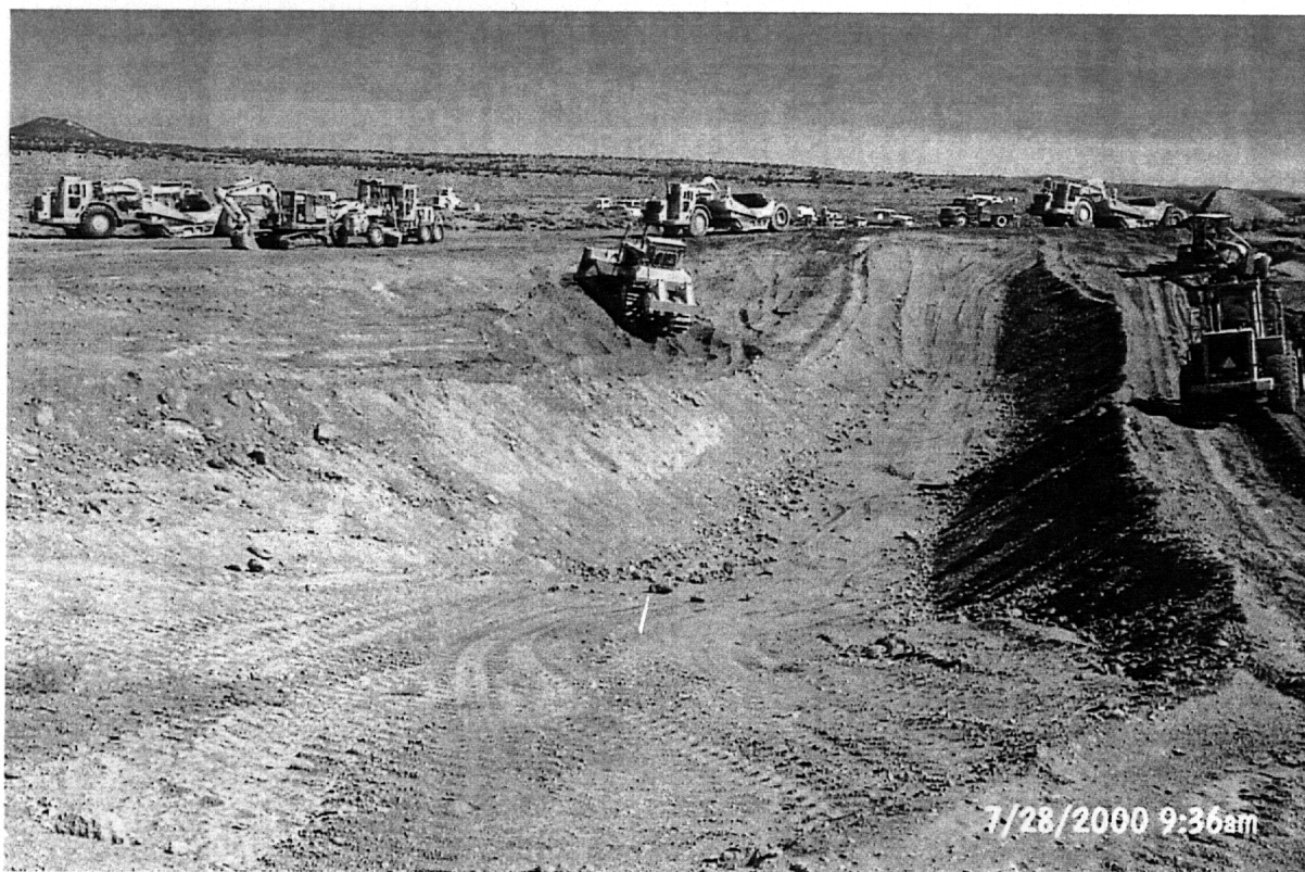
PHOTOGRAPH 6 - Excavation of the CMP Mud Relocation Trench
