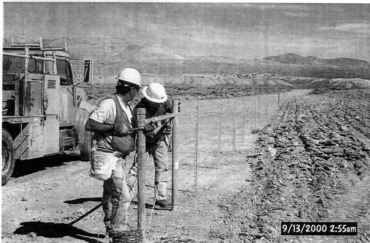
PHOTOGRAPH 17 - Erecting the CMP cover fence
