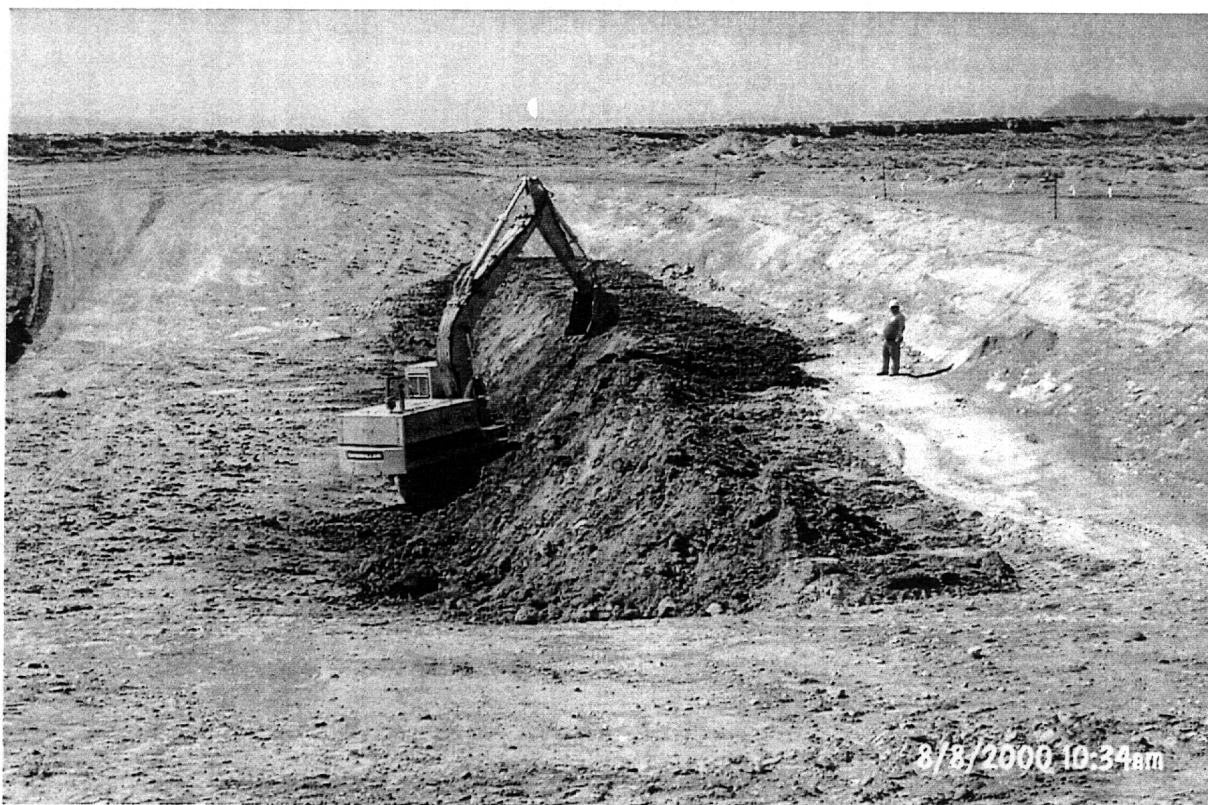
PHOTOGRAPH 10 - Leveling drilling material surface with Track Hoe
