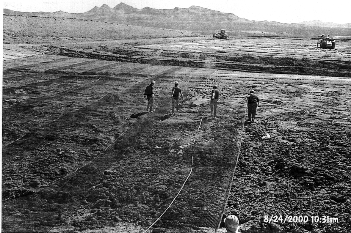
PHOTOGRAPH 13 - Placing geogrid over CMP Mud Relocation Trench
