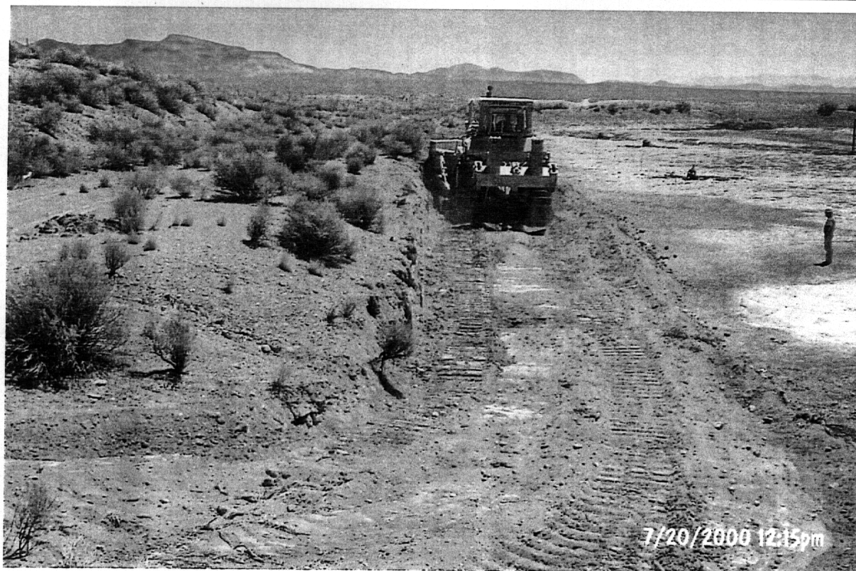
PHOTOGRAPH 1 - Cutting geogrid anchor bench for Central Mud Pit
