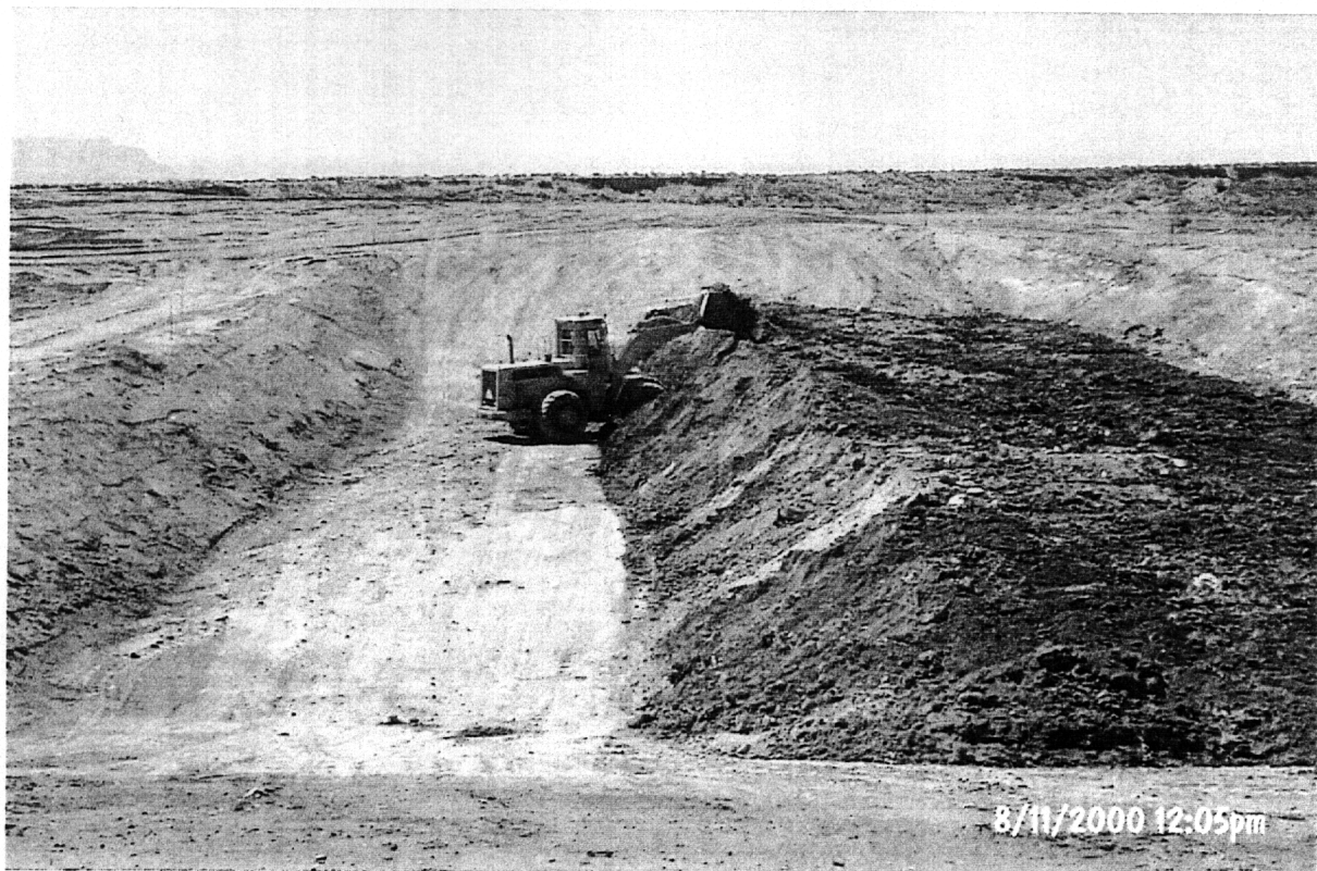
PHOTOGRAPH 9 - Stacking drilling material in the Mud Relocation Trench
