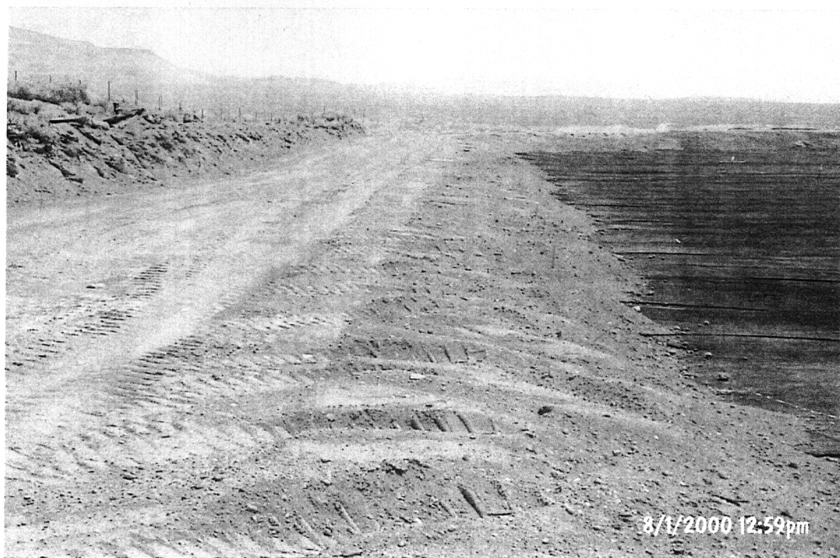
PHOTOGRAPH 3 - Geogrid anchored in place on CMP
