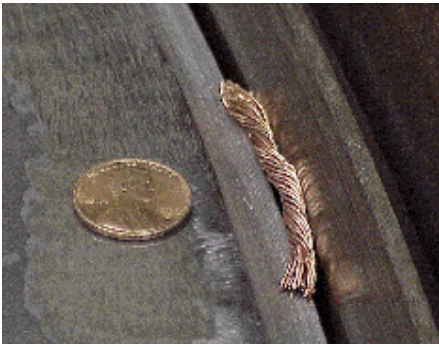
Fig. 2. Copper wire in joint
