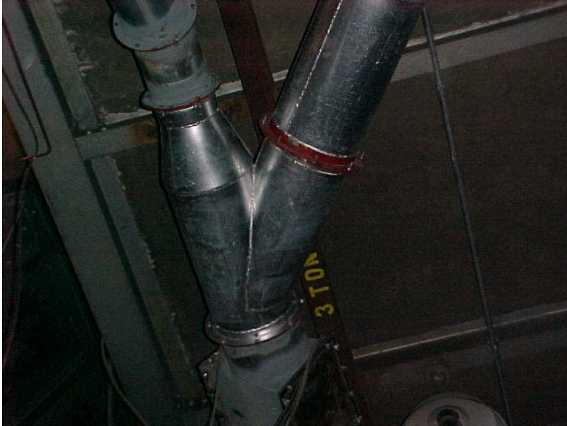
Figure 4-21. The Splitter for Transporting Switchgrass to Opposite Corners of #2 Boiler
