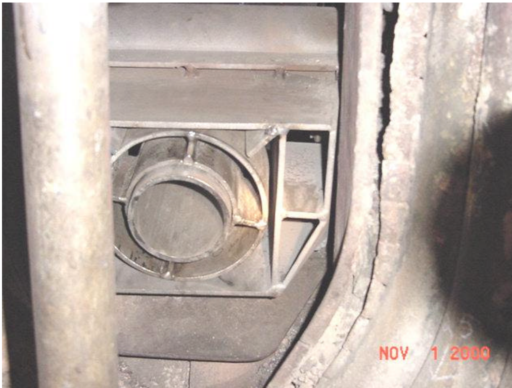
Figure 4-5. The Sawdust Injector in the Albright Boiler #3
