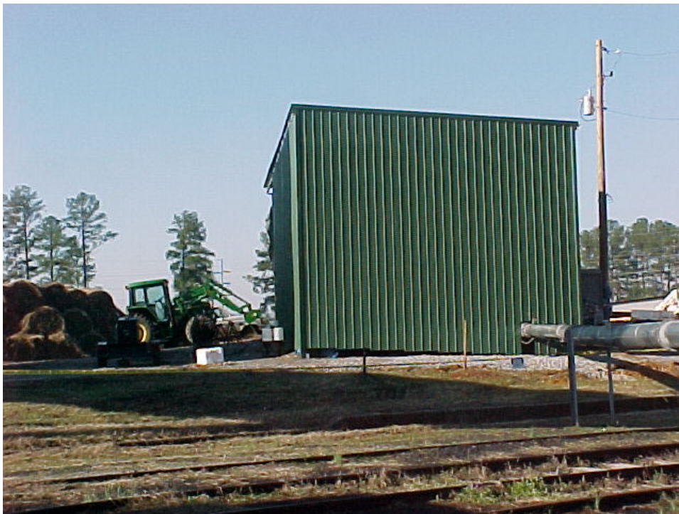
Figure S-11. The Switchgrass Cofiring Facility at Plant Gadsden with the Tractor Feeding a Bale, and the Pneumatic Transport Pipe Carrying the Switchgrass to the Boiler
