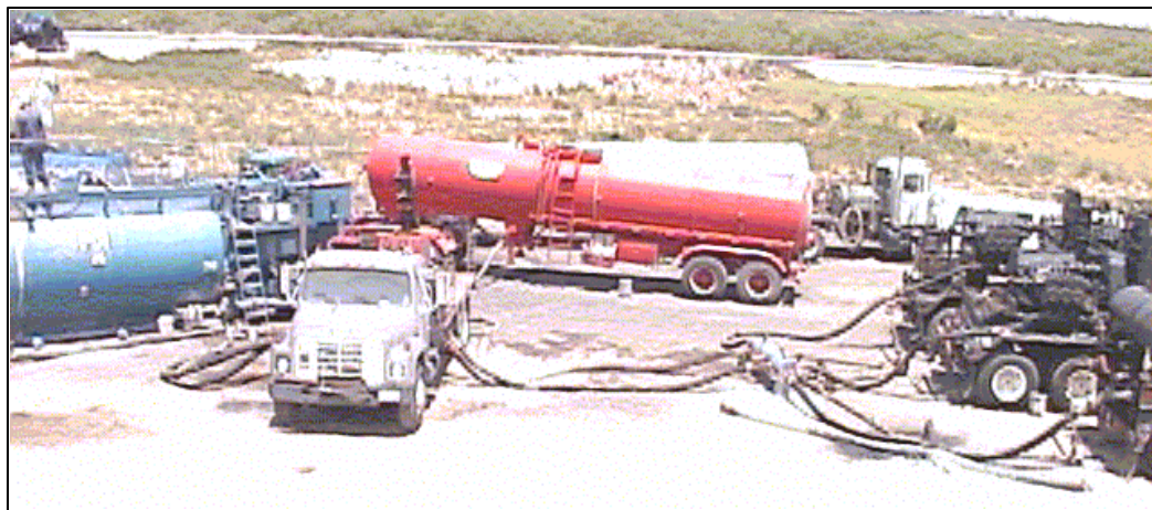
Figure 2. Mobile grout plant used for 1999 field demonstration.
