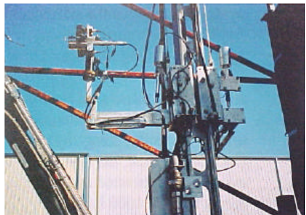
Figure 3. Camera assembly installed on mast.
