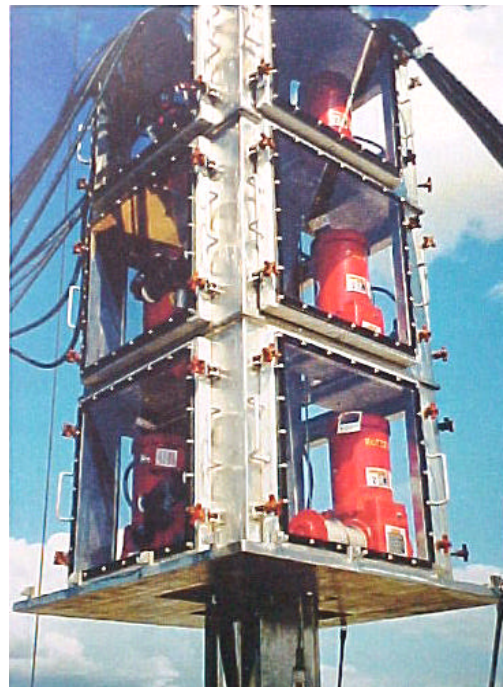
Figure 2. Winch stand assembly.
