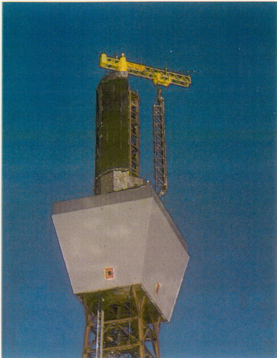
Figure 2-8. The Solar One Receiver Being Dismantled.
