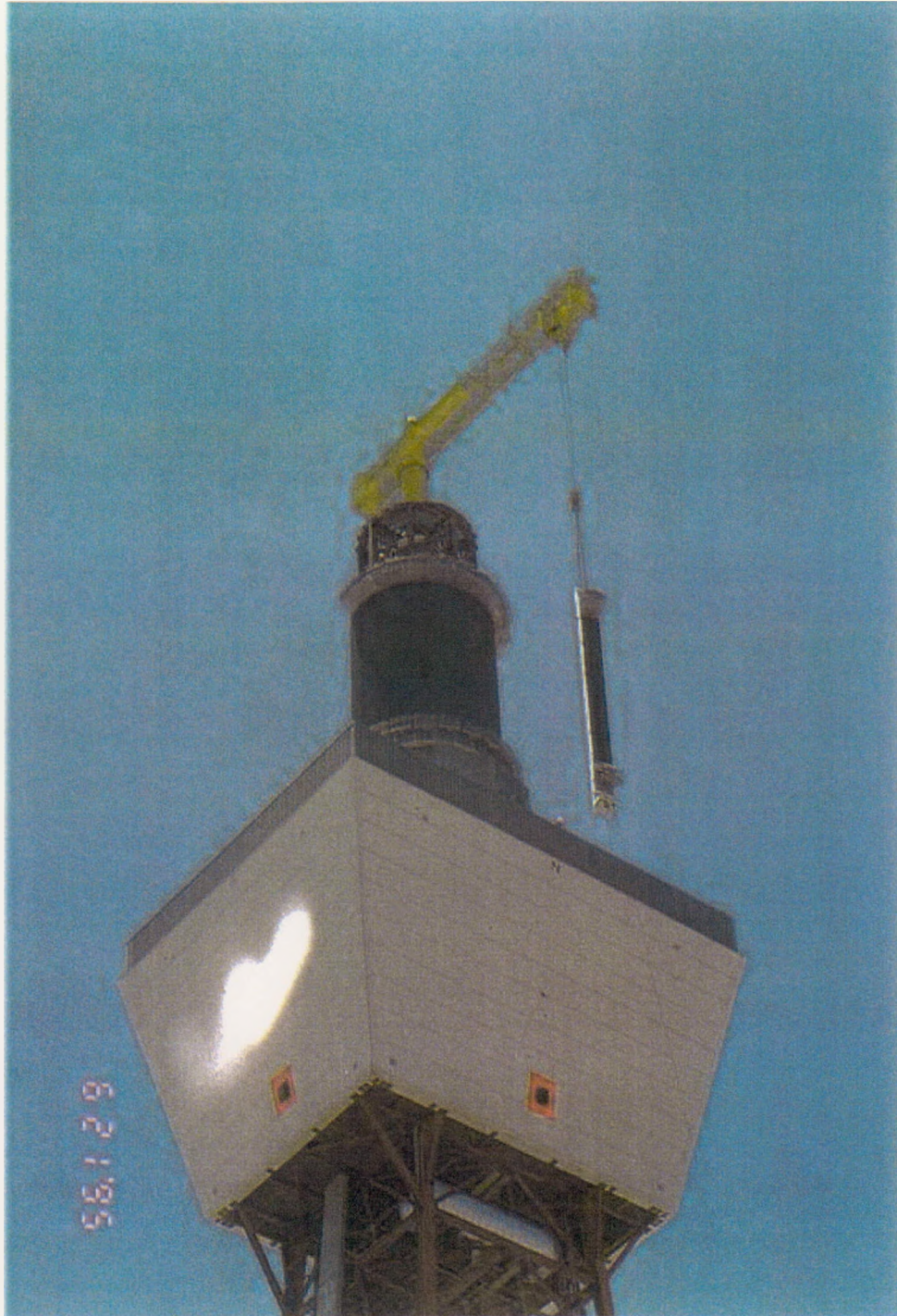
Figure 2-9. A Solar Two Receiver Panel Being Hoisted to the Top of the Tower.
