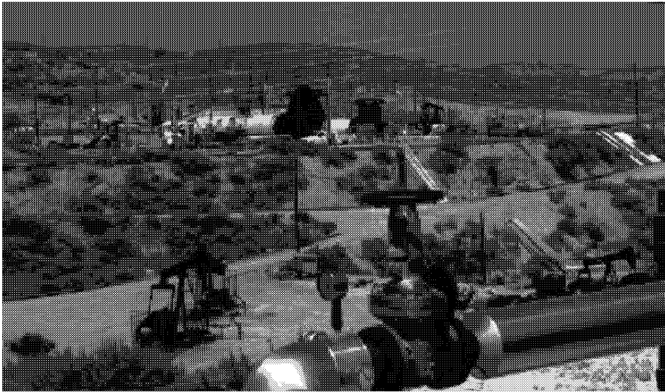
Figure 6-2: View north eastward across the entire 40 acre Pru Fee property. The Pru-209 producer is in the foreground. The white steam generators are near the center of the property.
