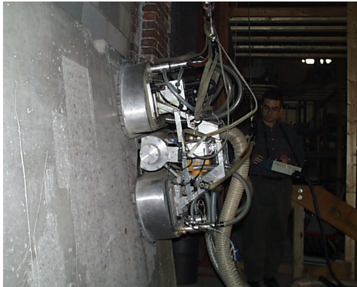
Figure 1 The IVOD system is used to decontaminate walls and ceilings.
