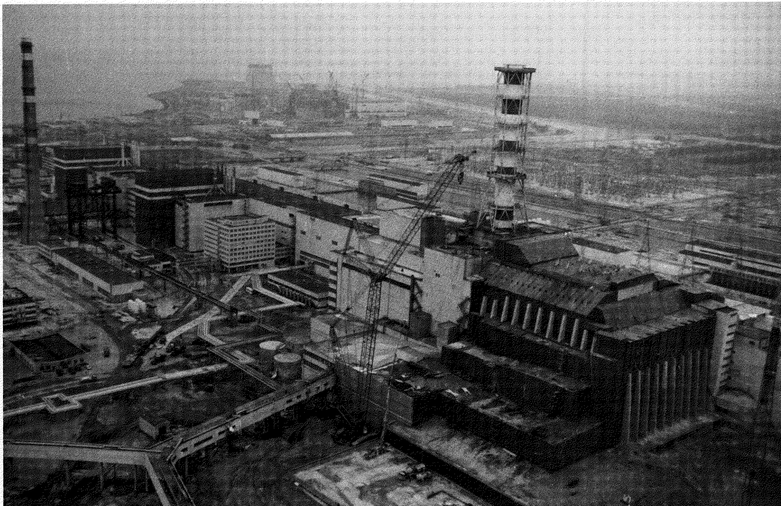
Fig. 2 Photograph of the nearly completed Chornobyl Unit 4 sarcophagus "Shelter" in November 1986 viewed from the northwest. (Photograph courtesy of Valentin Ivanovich Obodzinski of the Kurchatov Institute, Moscow.)
