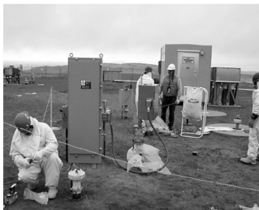
Field installation: Outdoor cabinet with probe and indoor cabinet
