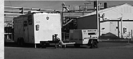
Control Trailer and Generator at Tank Farm
