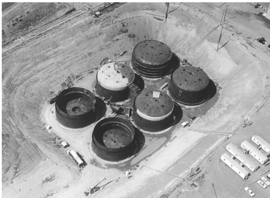
Figure 1.1. Double-Shell Tank Farm under Construction, circa 1980
